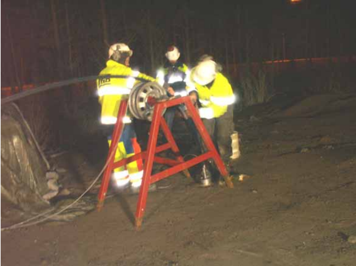
Figure 7. Installation of geofones in OL-PR10.
