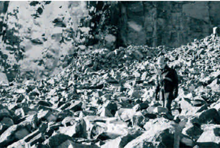
THE EXCAVATION OF ONKALO ALONE WILL GENERATE OVER 600 000 CUBIC METERS OF CRUSHED ROCK. THE TOTAL LENGTH OF THE ACCESS ROUTE, THE RESEARCH TUNNELS AND THE VENTILATION SHAFT IS OVER 8 KM.
