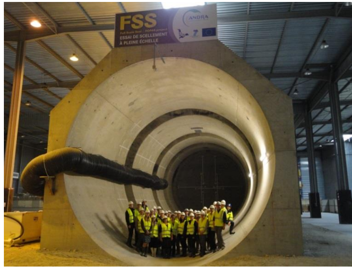
Fig.2: The FSS test box equipped with mine like ventilation before backfilling operations
