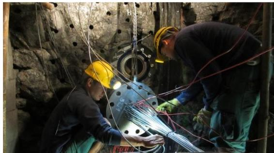
*Figure 7 - Cable head preparation*
