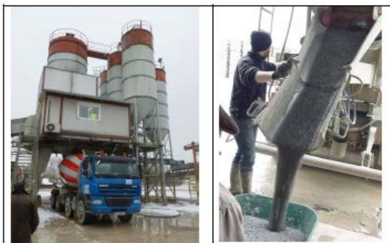
Figure 12: Concrete mixing plant & truck mixer (left) /sampling from the truck mixer (right)
