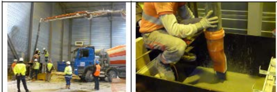
Figure 13: Truck mixer and pumping boom (left) & pouring inside metric cubic mold (right).
