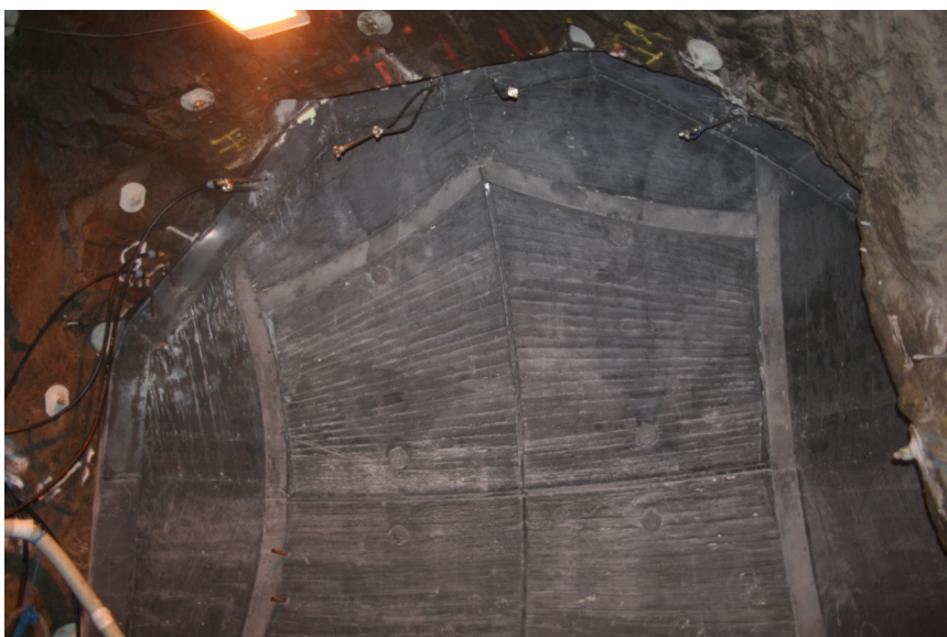
Figure 3. Experiment 3. DOMPLU plug 28 after plug casting. Photo:SKB.
