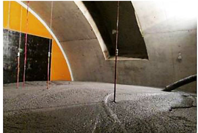
Casting of low pH concrete plug for the containment wall © Andra
