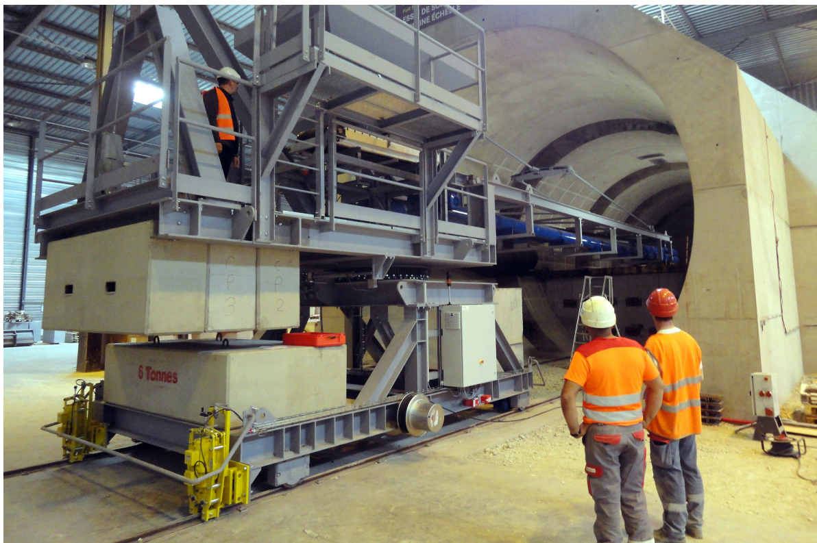
FSS test: Bentonite materials emplacement machine to be used for the construction of the swelling clay core. © Andra
