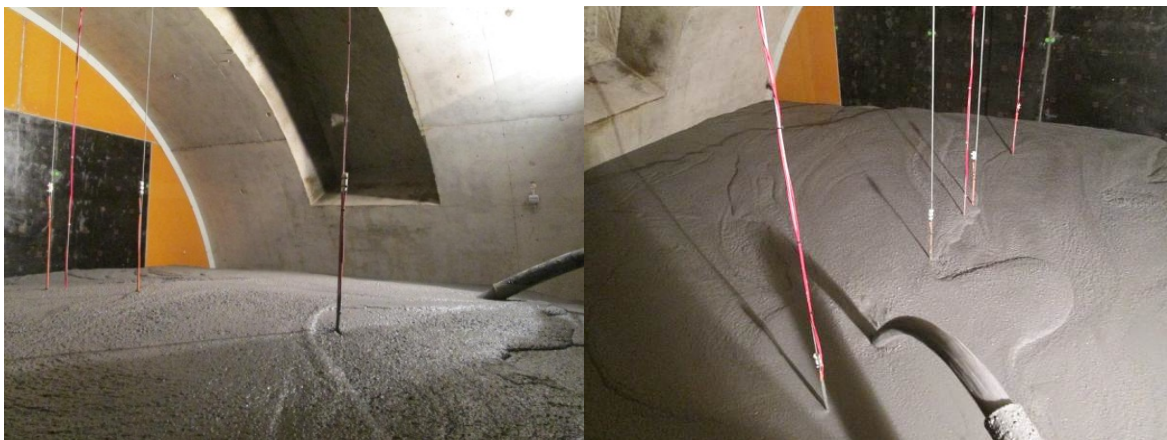
Figure 13: Pouring and even emplacement of SCC inside the test box
