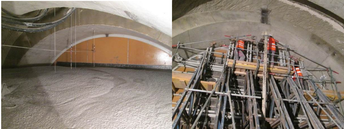
Figure 14: Emplacement of SCC close to the recess (left) and in the recess (right)
