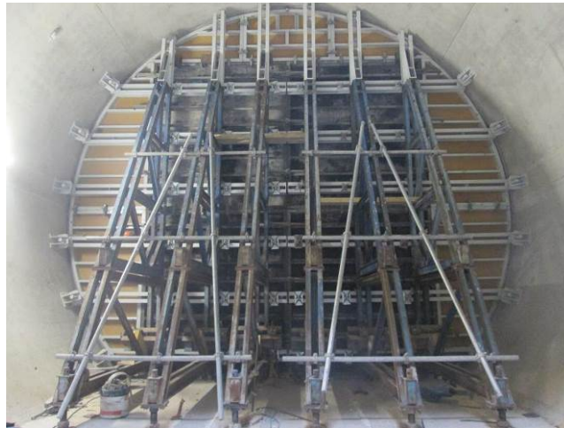
Figure 8: The one face circular formwork as erected
