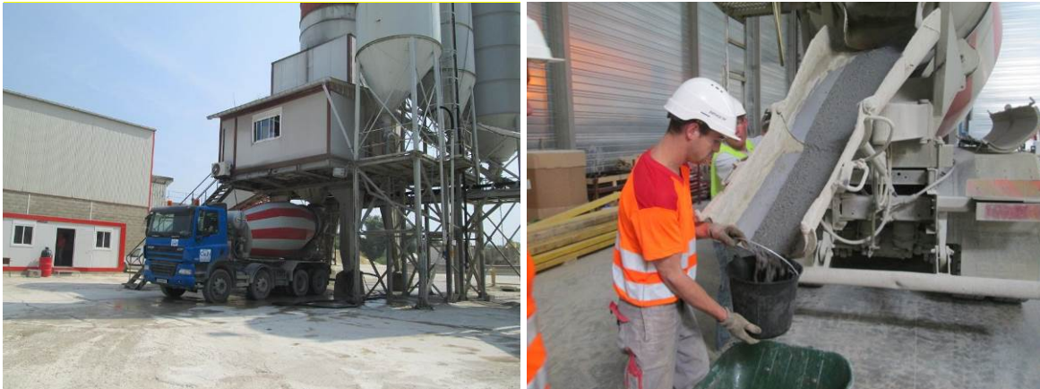
Figure 11: Preparation of concrete at the Saint-Dizier mixing plant (left) and concrete sampling at the FSS site (right)
