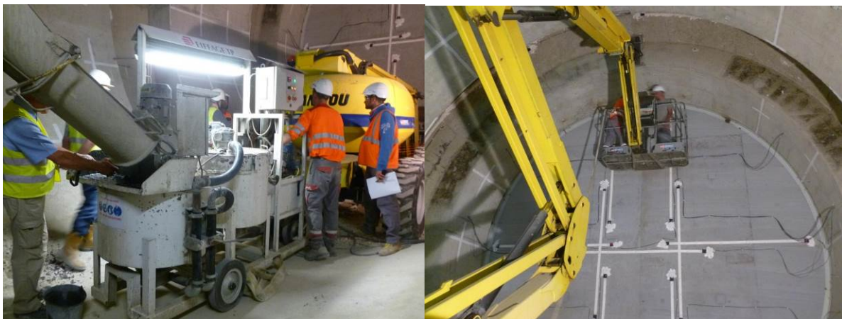
Figure 15: Injection of bonding grout at the summital contact between plug and box
