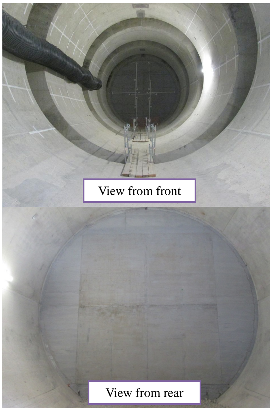
Figure 16: The SCC upstream containment wall as an end product
