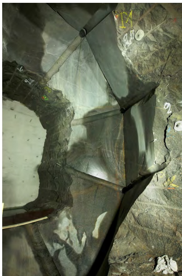
Fig 3. The excavated slot for DOMPLU
