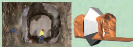
Careful rock excavation of the concrete dome abutment by the use of wire-sawing method
