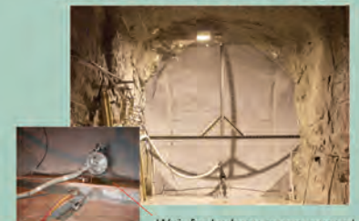
Weir for leakage measurement
