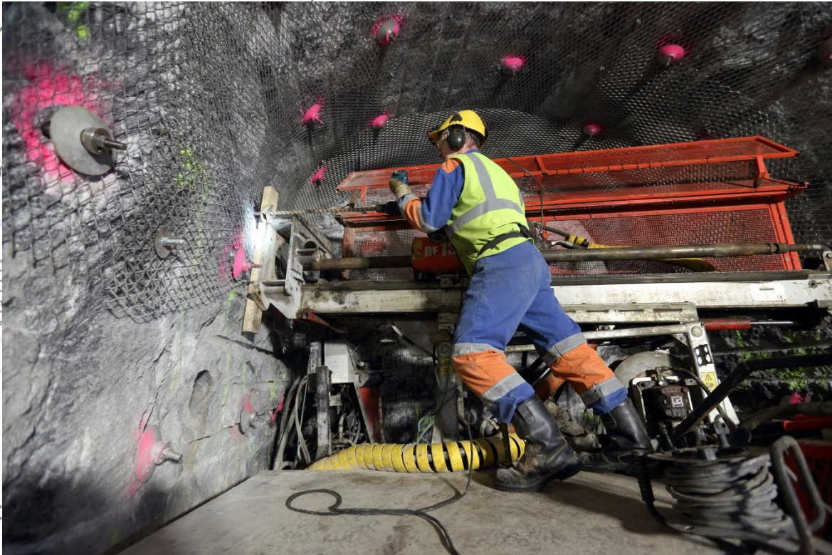
with concrete plug Drilling of lead-through pipes
