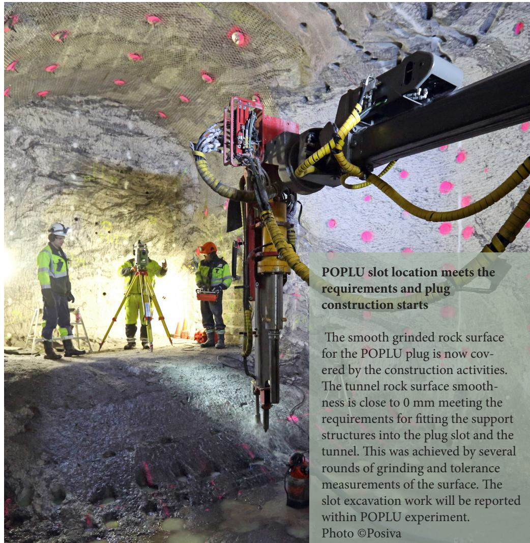
Photo from ONKALO demonstration area is showing slot excavation for the bottom section needed for construction of deposition tunnel plug. The POPLU Experiment is implemented in the future spent nuclear fuel disposal facility in Olkiluoto, Finland.
