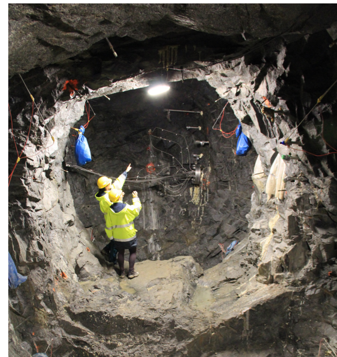
Tunnel is ready for emplacement actions. © CTU and SURAO
