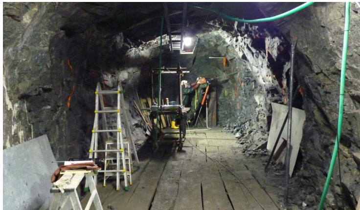
Figure 6 Grouting in niche SP-59
