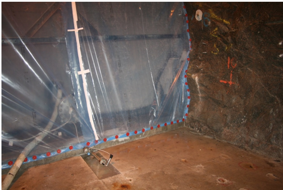
Figure 4-6. Installed plastic sheet, which encloses the concrete dome plug to prevent evaporative water loss.
