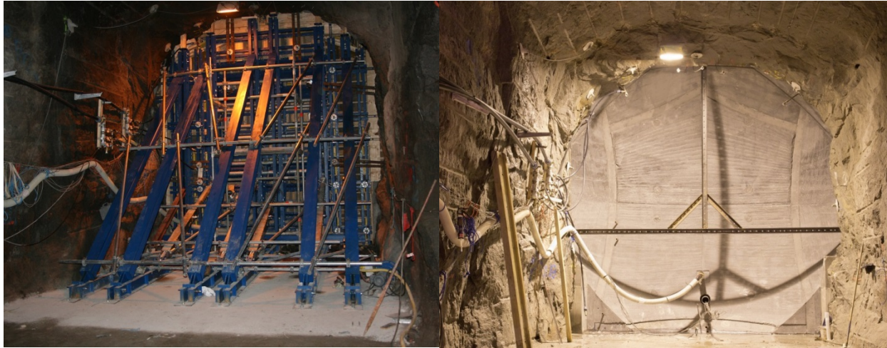
Figure 4-3. Left: Formwork by Doka used for casting of the concrete dome in March 2013. Right: The concrete dome after removal of formwork in late April 2013. The beam in front of the dome was used for positioning of displacement sensors.
