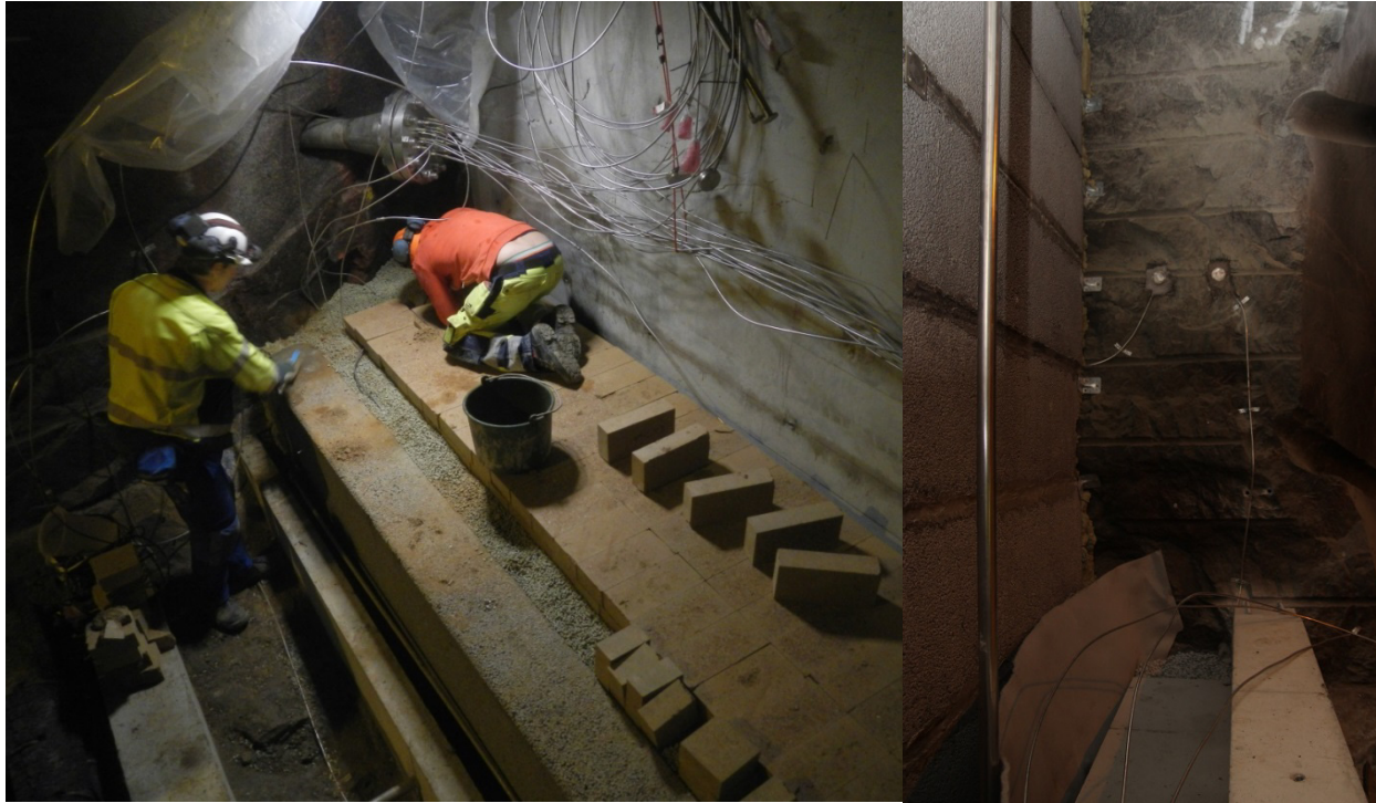
Figure 4-2. Photos of the DOMPLU installation in January 2013. Left: Top view of the arrangement of bentonite blocks and pellets in the backfill transition zone. Right: Side view of the filter section (LECA beams, drainage/air pipe and gravel), geotextile delimiter, bentonite seal (MX-80 blocks and pellets) and concrete beam delimiter. All cables inside the plugged volume are led in steel tubes to protect them from being damaged due to high water pressure.
