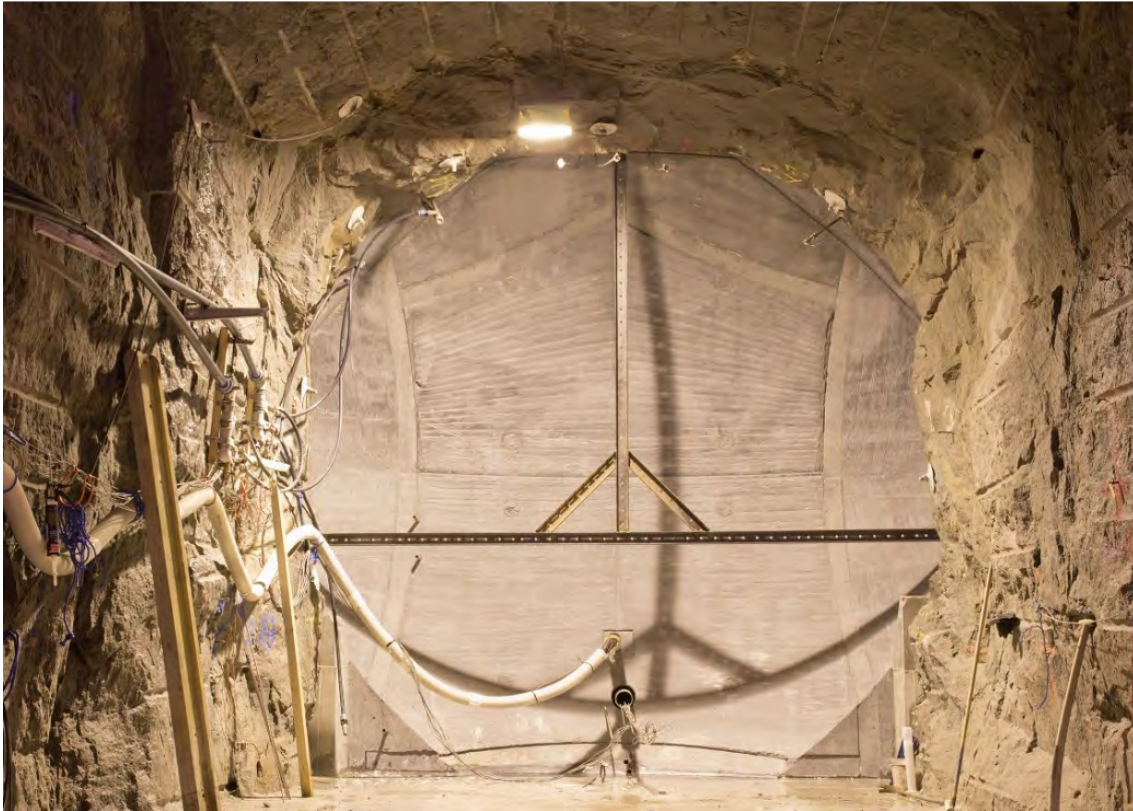
Figure 6-28. Photo of the cast concrete dome. The steel bars in front of the dome were later used for positioning of displacement sensors.
