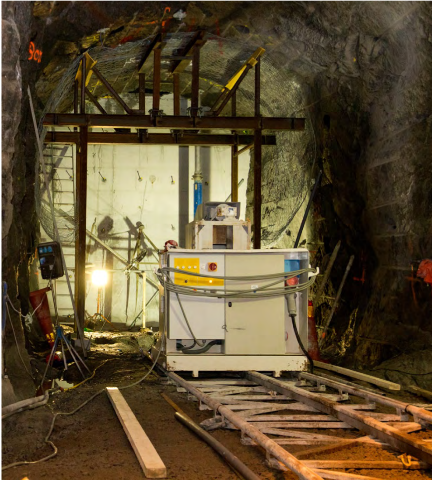
Figure 3-10. Wire-sawing equipment moving on rails in TAS01.
