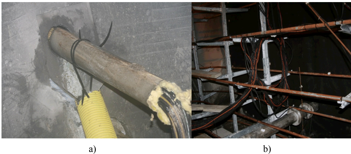
Figure 9-53. Located leakage through the cable bundle for sensors installed in the concrete dome.
