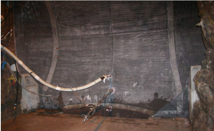
Figure 7-11. Lead-through in the concrete dome. The upper is for cables of measurement equipment installed inside the concrete dome and the bottom is for equipment installed in the bentonite seal and in the slot (i.e. not those cast inside the concrete dome).
