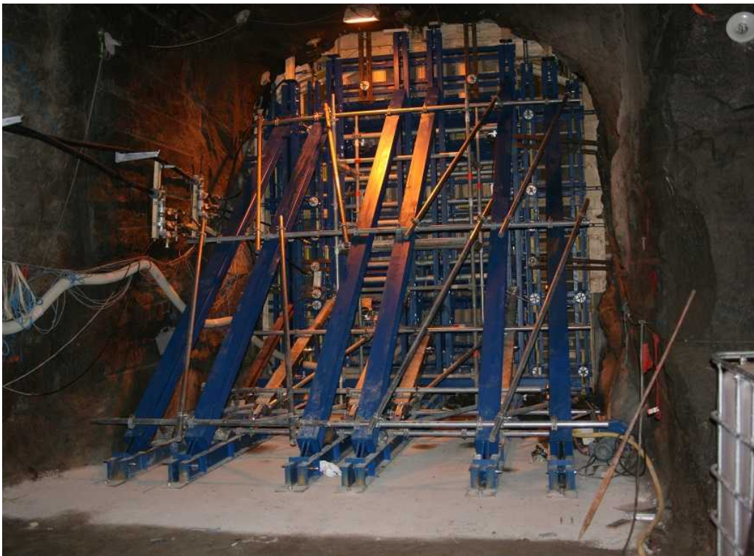
Figure 6-25. Concrete formwork with supporting struts to transfer the hydrostatic pressure from the concrete slurry to the surrounding rock.
