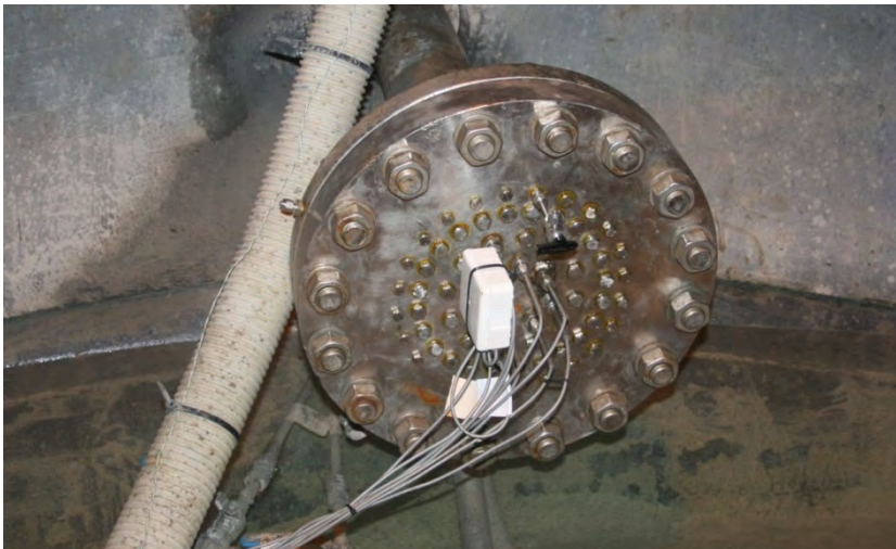
Figure 7-12. Lead-through in the concrete dome, intended for cables of measurement equipment installed in the bentonite seal and in the slot (i.e. not those cast inside the concrete dome). Here also shown with the water tight connection.
