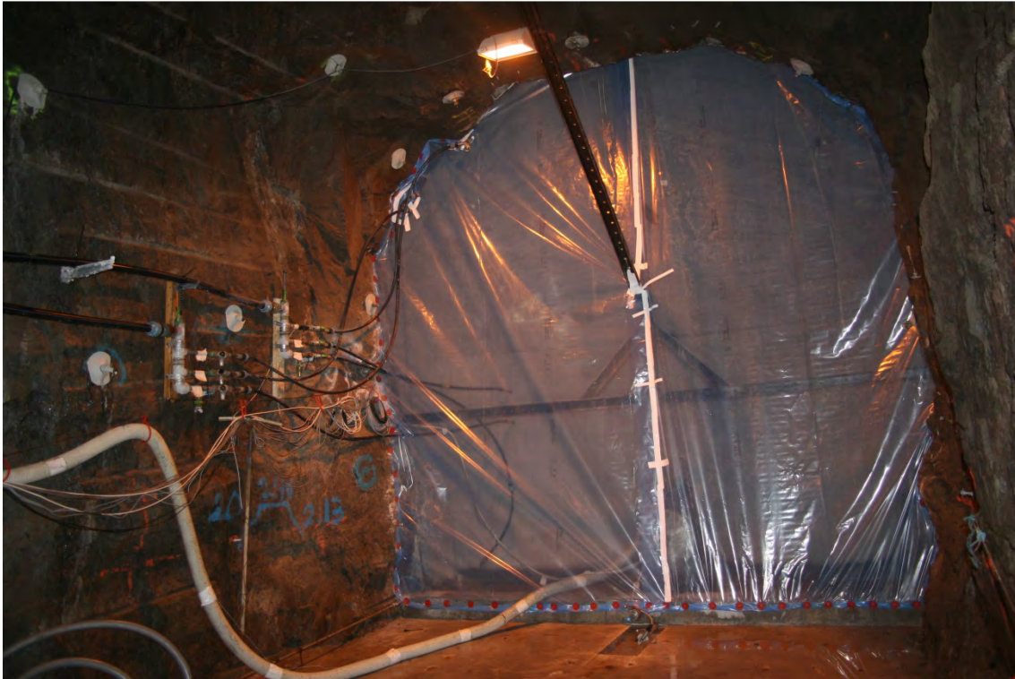
Figure 6-31. Installed plastic sheet, which encloses the concrete dome plug to prevent evaporative water loss.
