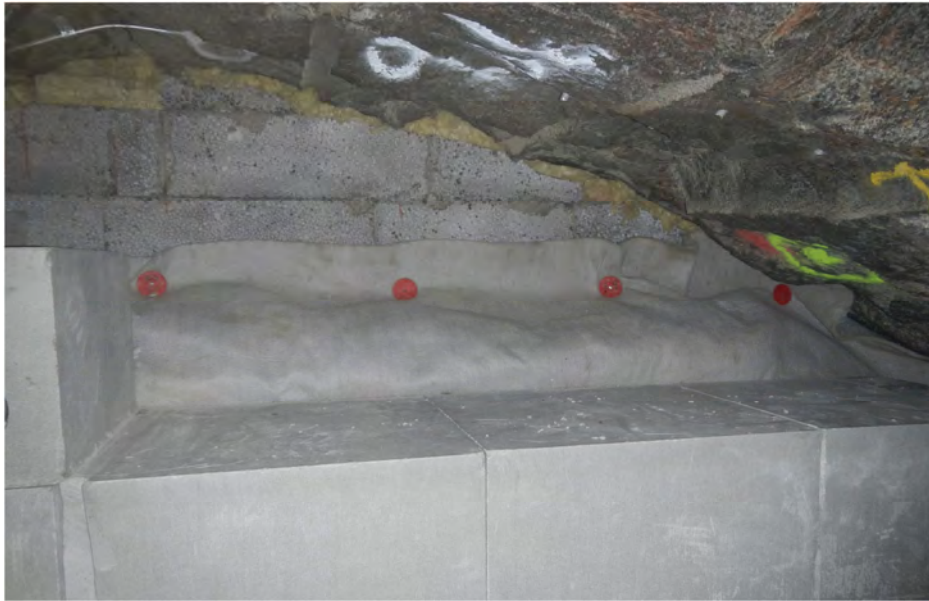
Figure 6-32. Photo showing the space left above the gravel section. The geotextile was folded in over the uppermost gravel surface.
