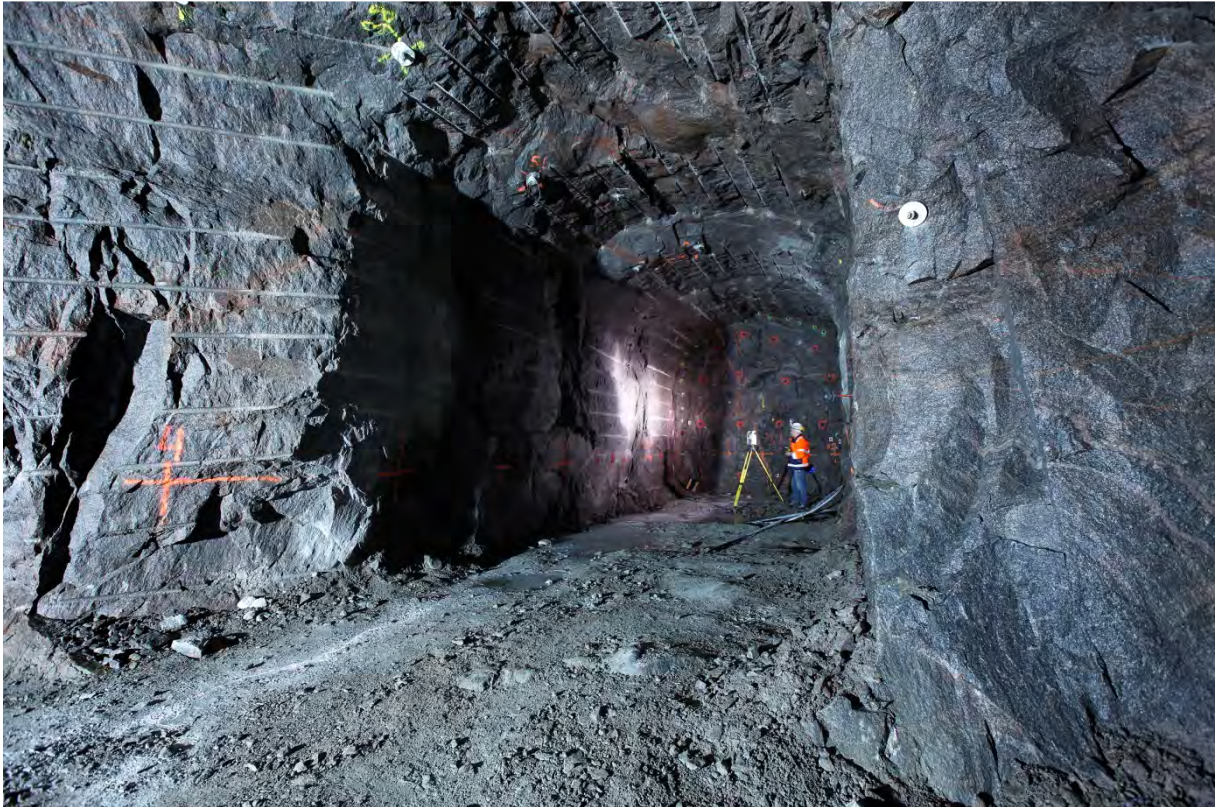
Figure 3-6. Photo of the completed test tunnel TAS01. Geodetic survey is ongoing to mark out positions of the plug components.
