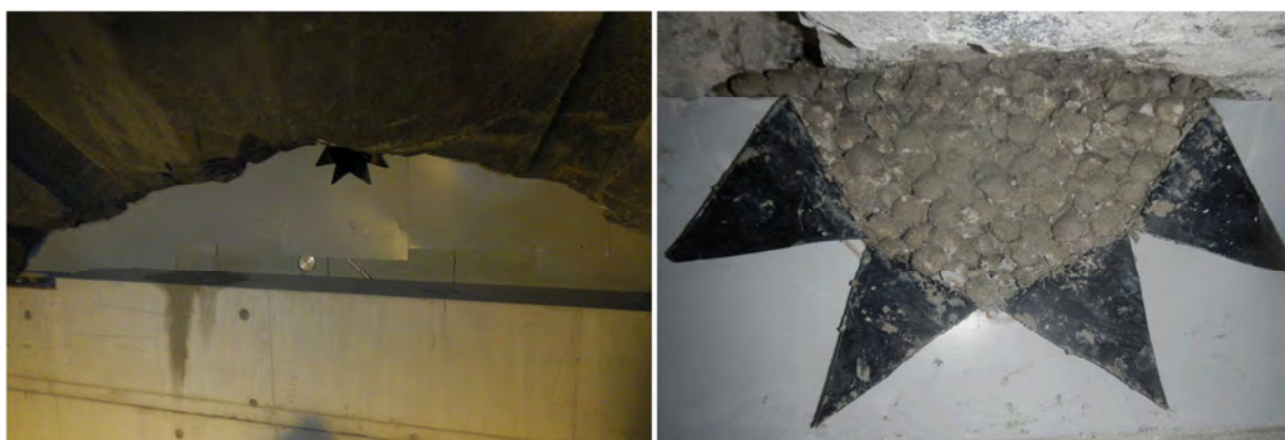
Figure 6-34. Left: Photo showing the steel plate fastened against the uppermost row of bentonite blocks Right: Close-up showing the opening through which the last pellets were installed.
