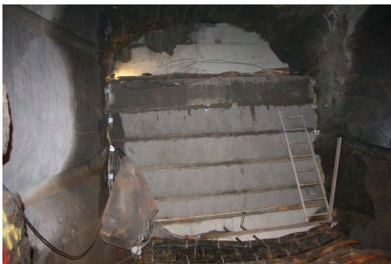
Figure 6-9. Installation of the LECA beams.
