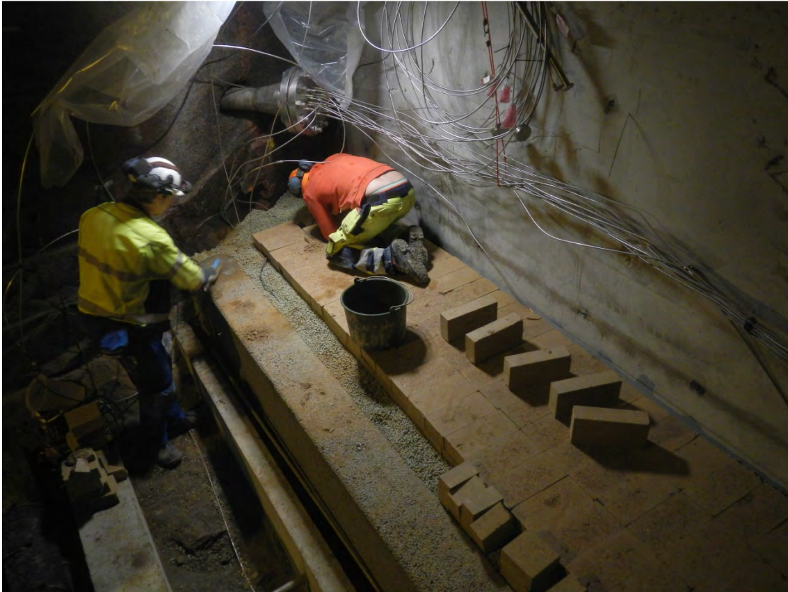
Figure 6-5. View of the arrangement of bentonite blocks and pellets in the backfill transition zone for DOMPLU.
