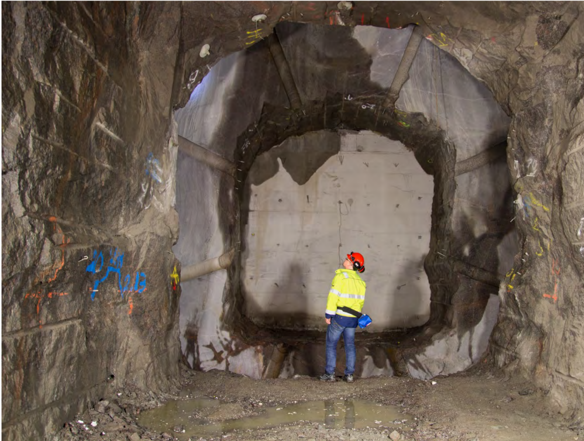
Figure 3-11. TAS01 with the excavated slot abutment for the concrete dome.
