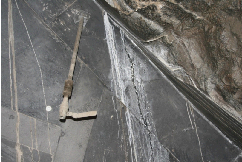
Figure 9-50. Observed water leakage in the interface between the concrete dome and the rock, in the top of the slot (at 13 o'clock). Note that the dark line on the face of the dome is water not a crack in concrete.
