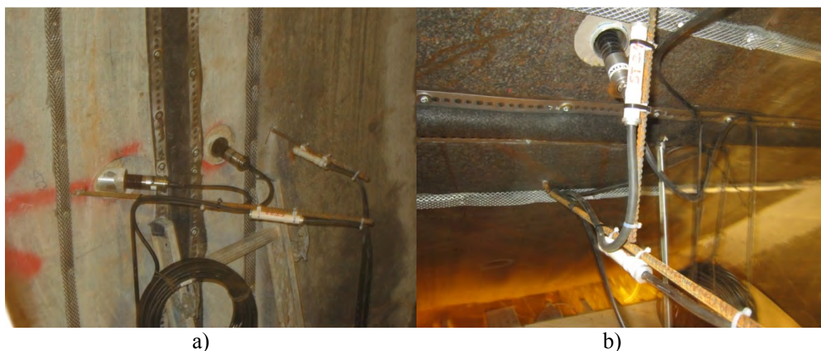
Figure 9-42. Photo of the two strain gauges ST23, (Figure (a)) and ST25 (Figure (b)) that failed during contact grouting.
