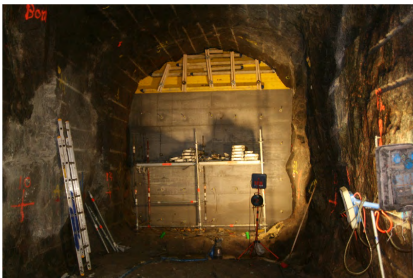
Figure 6-2. Photo of the concrete wall during removal of the formwork subsequent to casting.
