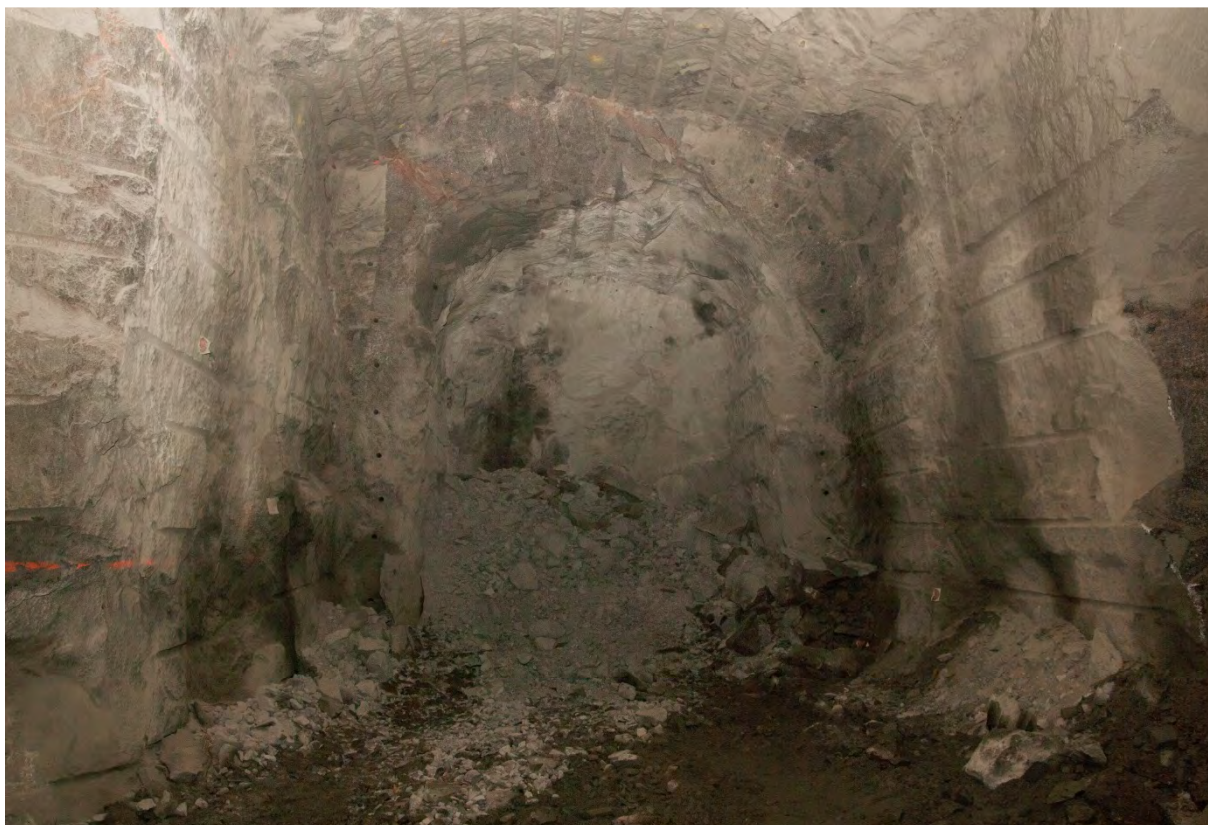
Figure 3-5. Photo of the test tunnel TAS01 during ongoing excavation of the third round. The perimeter boreholes to be used for separate charging and blasting of the peripheral tunnel contour are visible.
