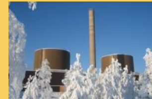
Loviisa power plant (LO1-2)
