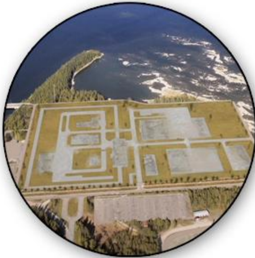
Construction around 10 years
