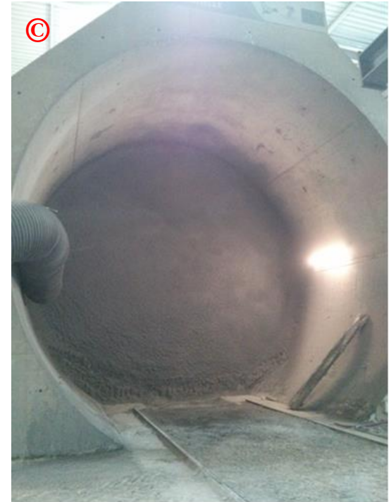
End of construction
