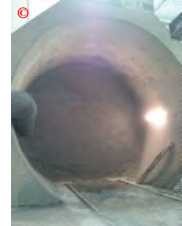
End of construction
