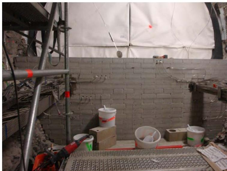
Fig. 2.5 General layout of the NSC experiment in the MHM-URL and seal construction in the drift using bentonite-sand blocks and bentonite pellets /DEL 15/
