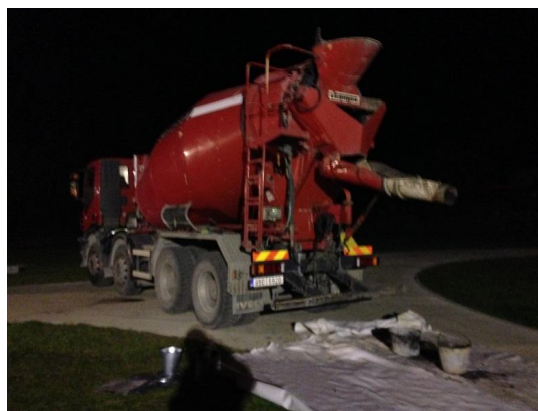
Figure 1: Concrete truck delivering concrete at the gallery entrance
