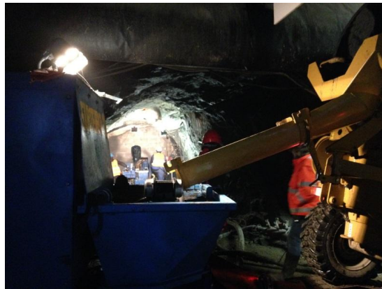
Figure 3: Transferring the concrete into the concrete pumps
