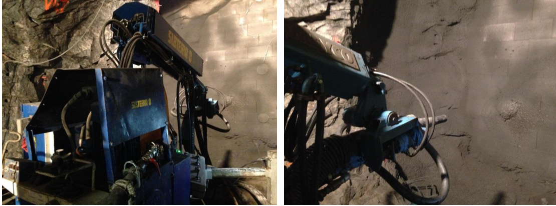
Figure 4: Shotcreting operations
