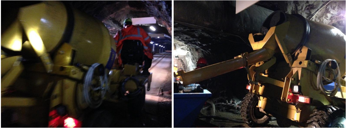
Figure 2: Transporting the concrete within the Joseph Gallery
