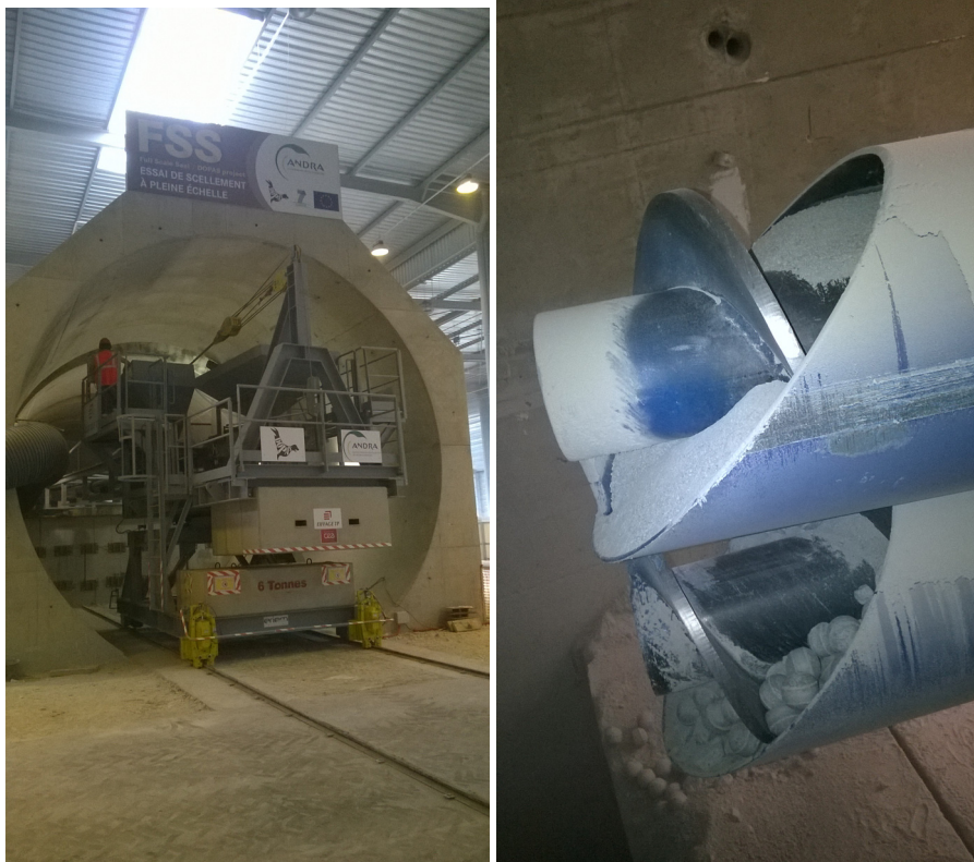
Figure 3: Bentonite materials transferred into filling machine and deposited into the core of the seal using augers.
