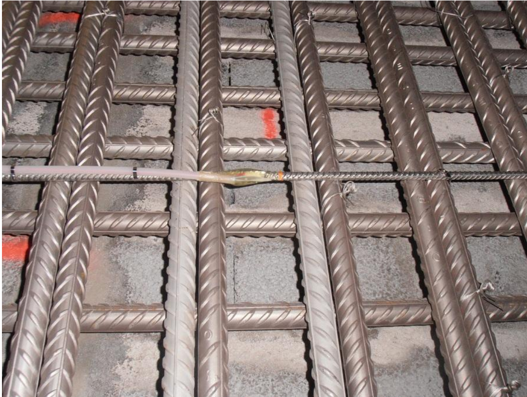
Figure 4.8 Strain gauge in place. Photo by Michal Roll.
