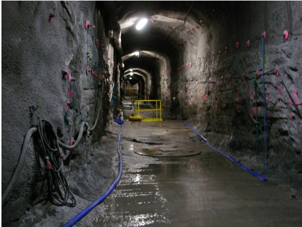
Figure 4.11 DT2 with test deposition holes and water as a result of leakage from fracture zone. Photo by Mark Crawford.
