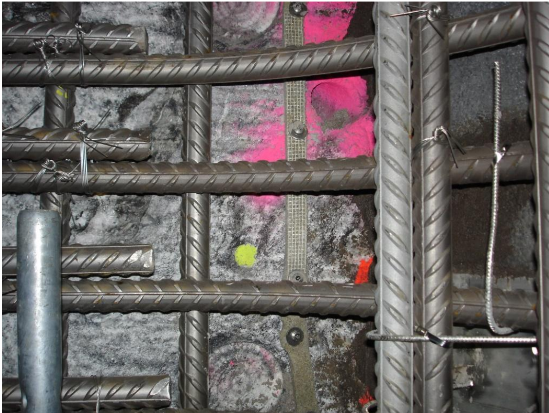
Figure 4.5 Close-up of stainless steel reinforcements, and bentonite tape attached to rock in the centre of the picture. Photo by Mark Crawford.
