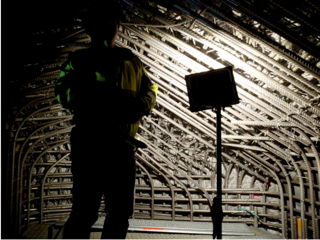
Figure 4.6 Structure of the top part of the plug from the inside, showing layers of reinforcements. Photo by Jo Smith.
