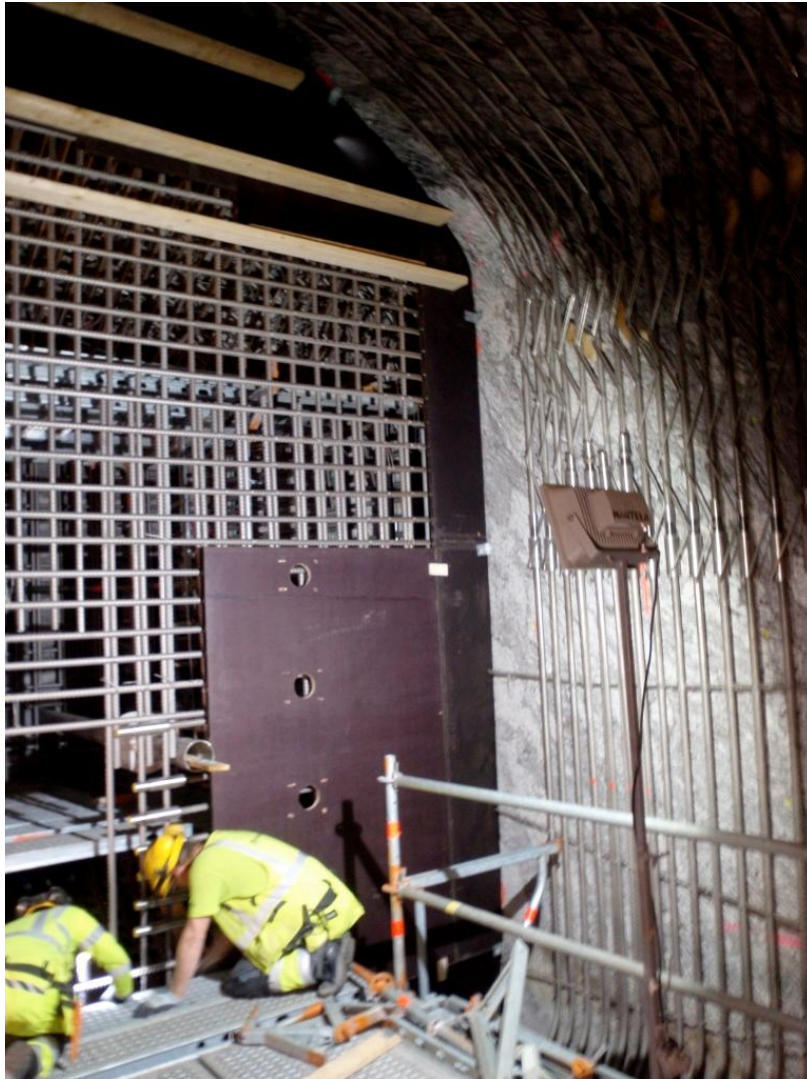
Figure 4.3 Front of the first part of the plug structure, showing stainless steel bar reinforcements, manhole in the bottom left for access to the plug interior, and formwork boards being fitted. Photo by Jo Smith.
