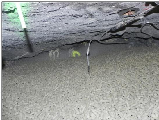
*Figure 21 - Upper part of the drift – the space intended for backfilling using spraying technology*
