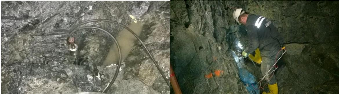
Figure 27 – Water pressure testing in the near-surface layer
