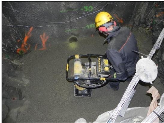
*Figure 20 - Pellet emplacement (compaction)*
