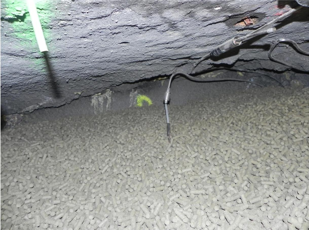
**Figure 38 - Upper part of the drift – space to be filled by spraying**
