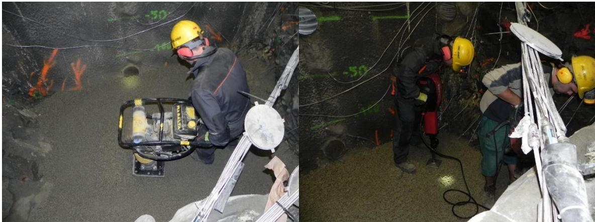
**Figure 36 - Vibration compaction**
