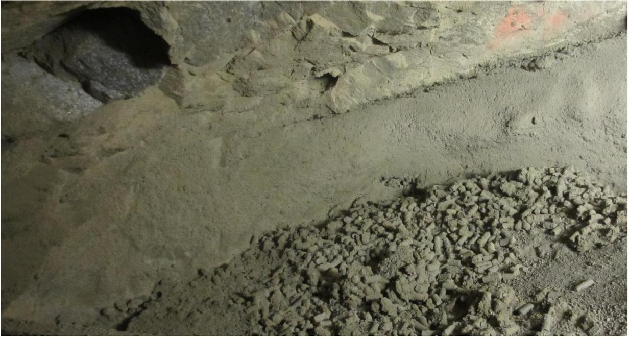
**Figure 40 - Sprayed bentonite**
