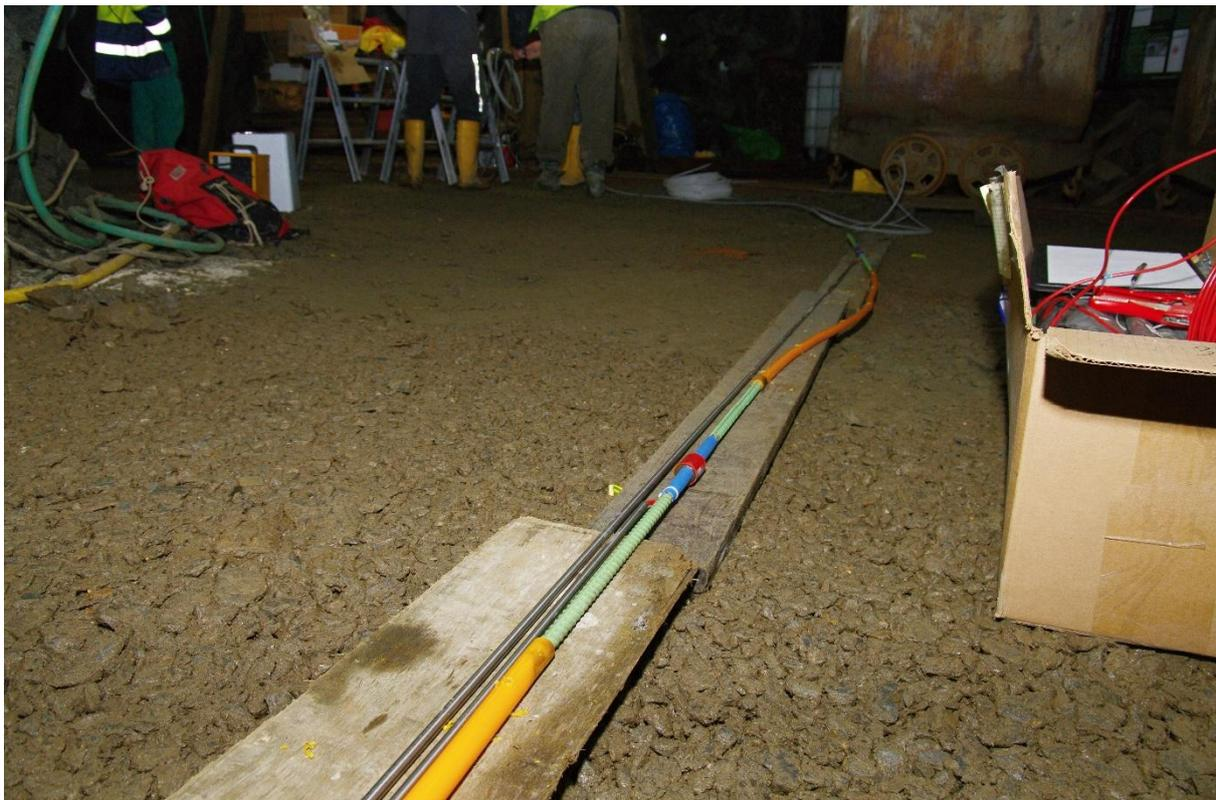
**Figure 24 - Rock bolt assembly prior to installation**
