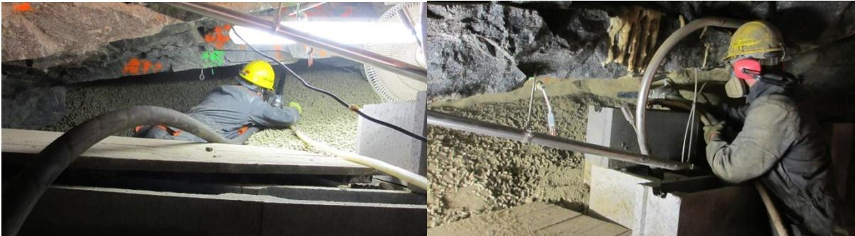
**Figure 39 - Spraying of the bentonite**
