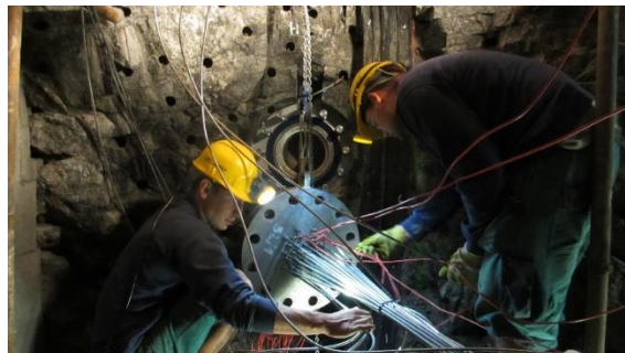
Figure 7 - Cable head preparation
