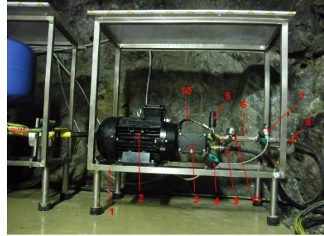
Figure 27 - High pressure unit
