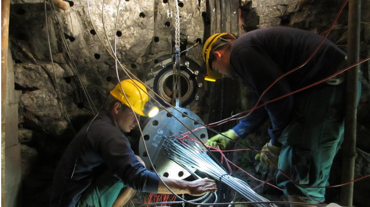
Figure 69 - Installation of cable head assembly B (June 2015)
