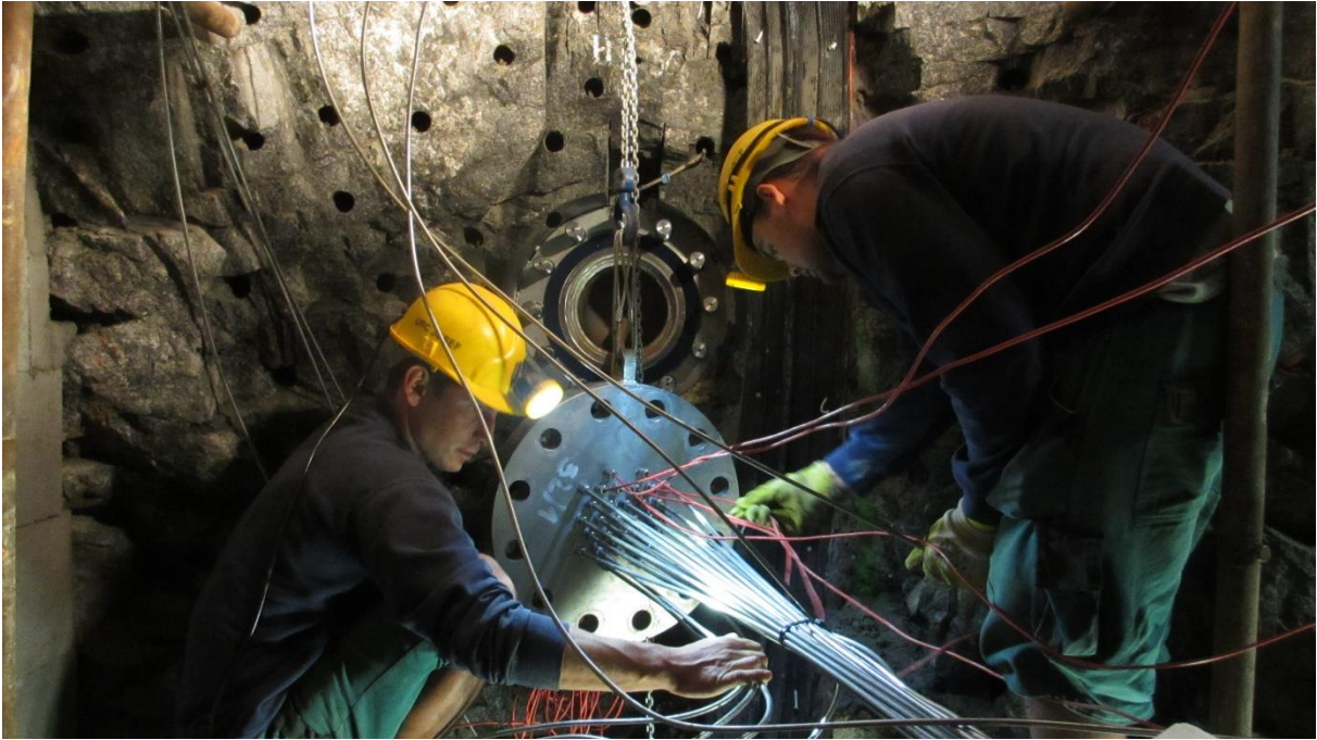
Figure 15 - Cable head preparation (outer plug, 17 June 2015)
