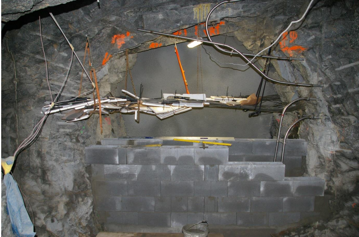
Figure 66 - Cable head assemblies installed, 1 st part of the filter separation walls erected, pressurisation tubing into the filter installed (December 2014)
