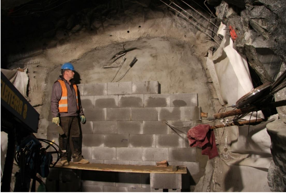
Figure 13 - Separation wall erection (4 November 2014)
