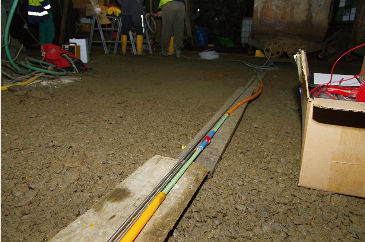
Figure 59 - Rock bolt assembly prior to installation
