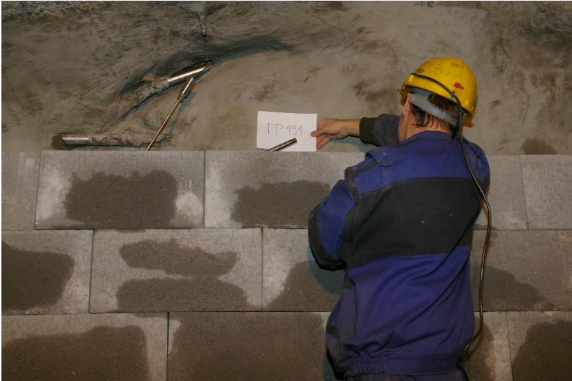
Figure 63 - Piezometer installation in the pressurisation chamber
