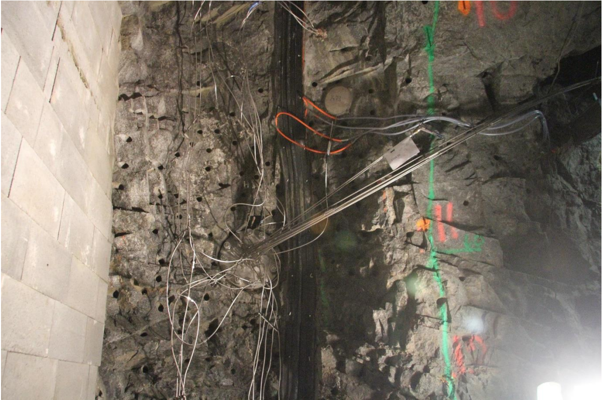
Figure 16 - Cable head and instrumentation before shotcreting (outer plug, 19 June 2015)
