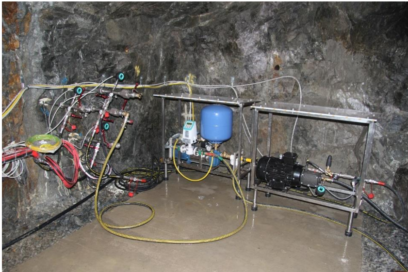
Figure 29 - Technological equipment installation in the niche (24 February 2015)
