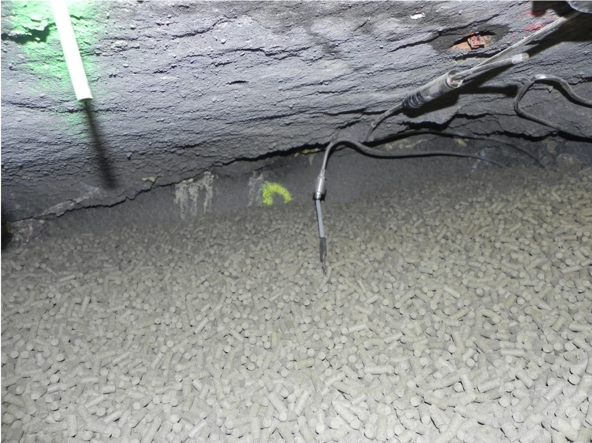
Figure 41 - Upper part of the drift – space to be filled by spraying
