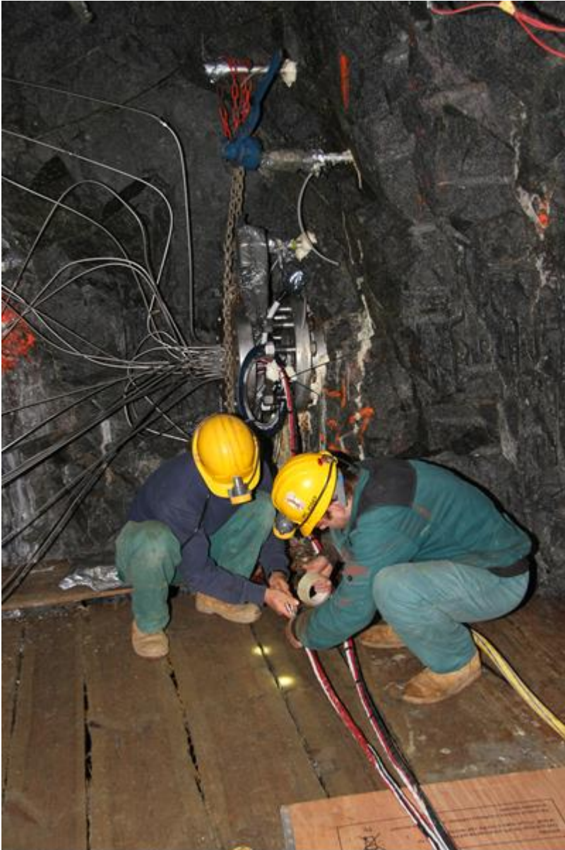
Figure 6 - Preparation for the leading of the cables
