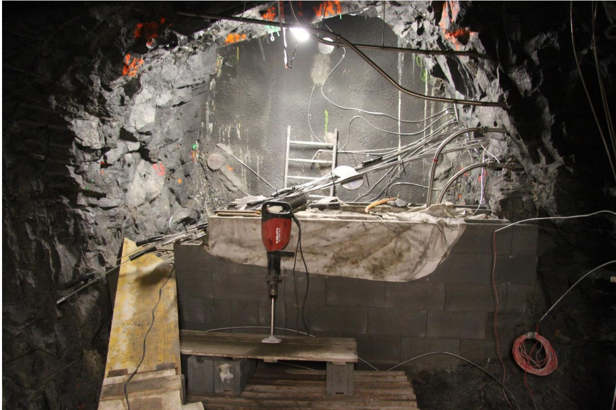
Figure 24 - First part of the filter erected (photo taken at the time of the start of bentonite installation, 5 June 2015)
