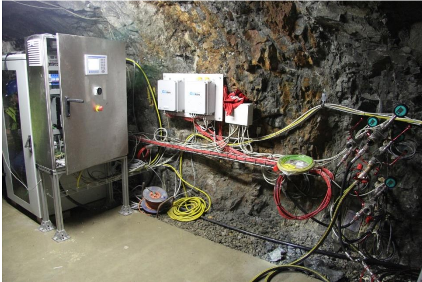
Figure 28 – Technological equipment installation in the niche (24 February 2015)
