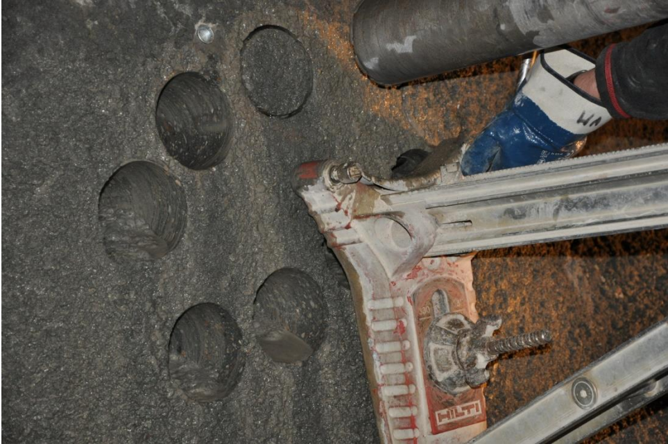
Figure 17 - Core sampling in-situ (material qualification test)
