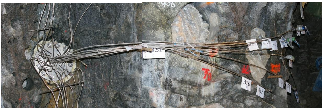
Figure 65 - Sensors temporarily stored on the side of the niche
