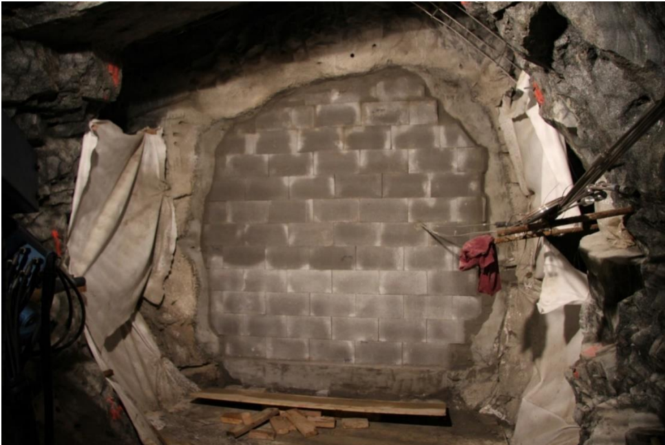
Figure 14 - Completed separation wall (5 November 2014)
