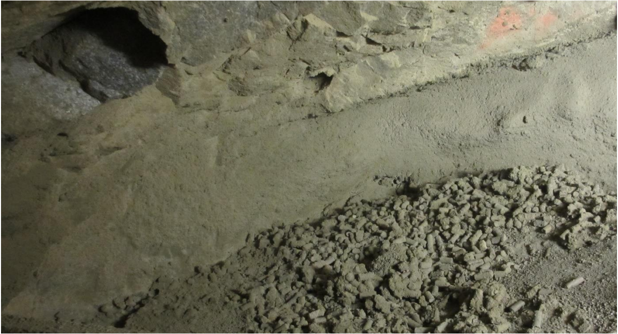
Figure 43 - Sprayed bentonite
