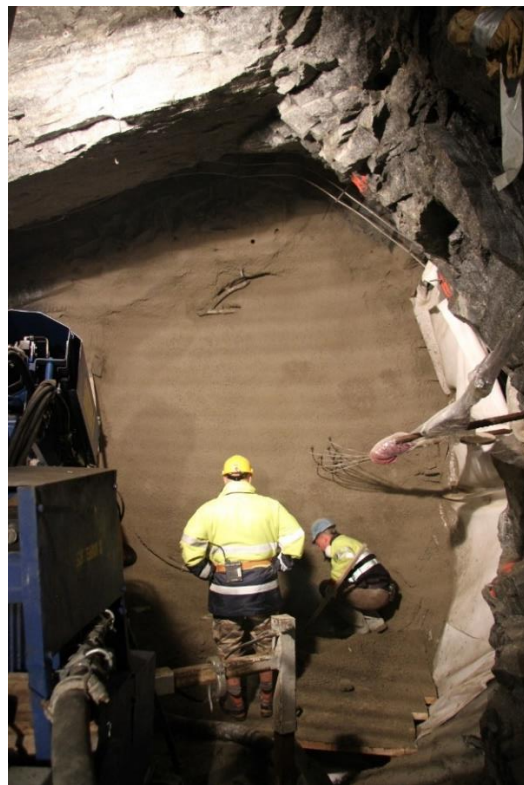
Figure 12 - Completed shotcreting (27 October 2014)
