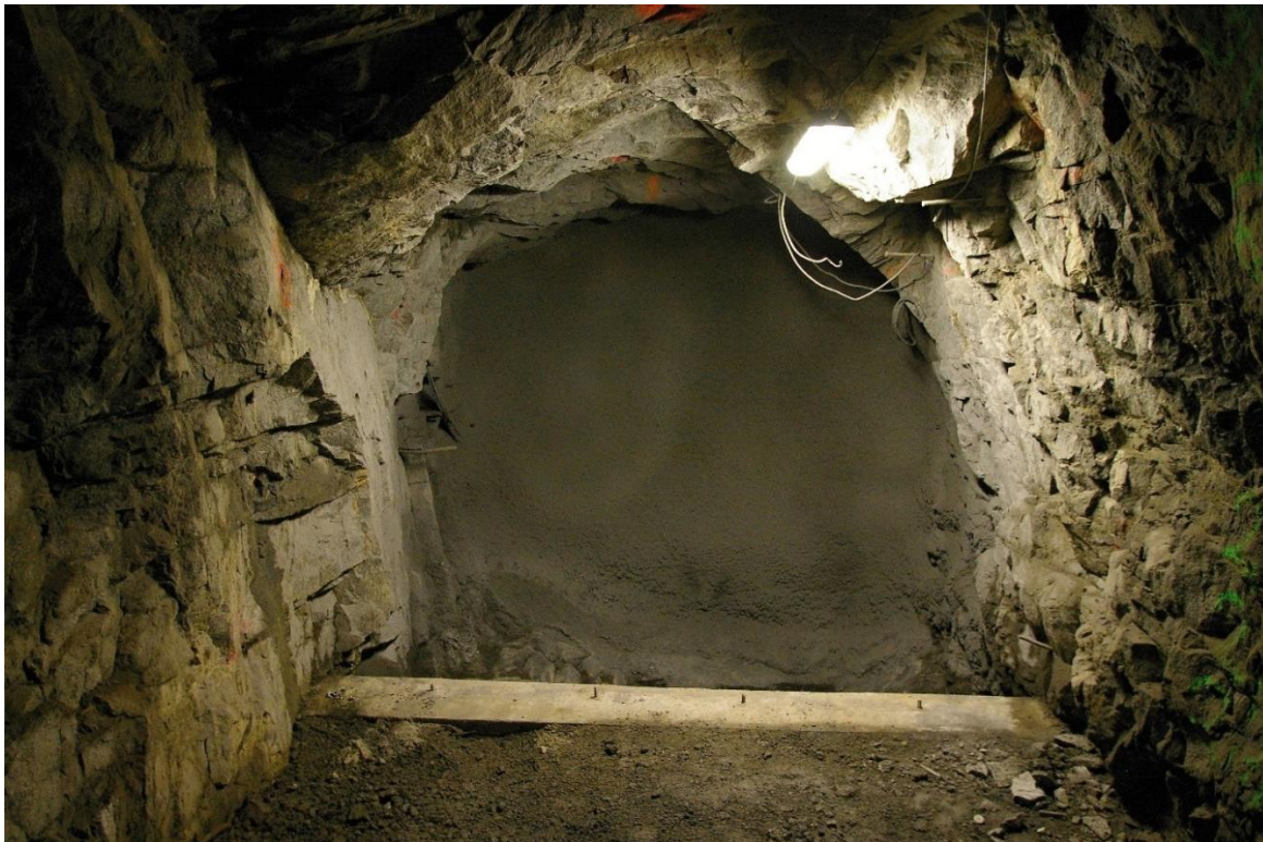
Figure 20 - Finished outer plug
