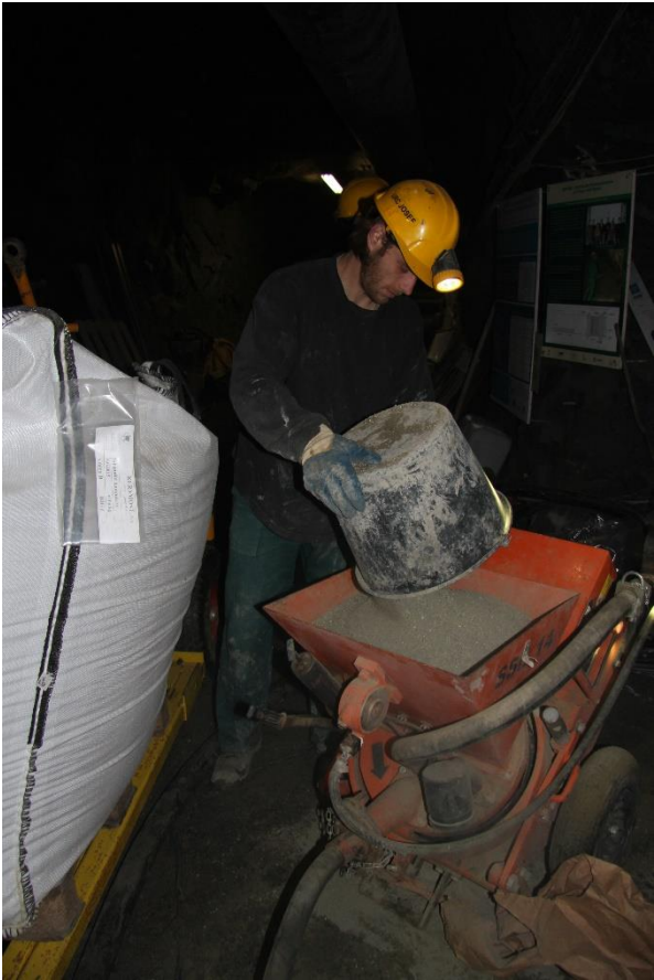
Figure 44 - Spraying machine
