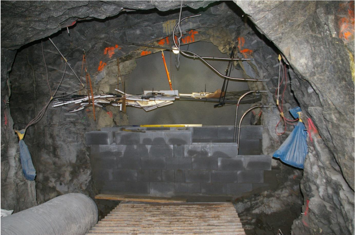
Figure 23 - Lower part of separation wall erection with the installed pressurisation piping (5 December 2014)
