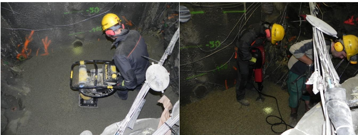
Figure 39 - Vibration compaction
