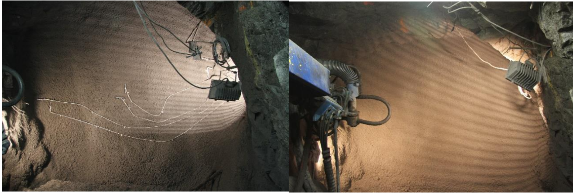
Figure 19 - Outer plug erection (19/20 June 2015)
