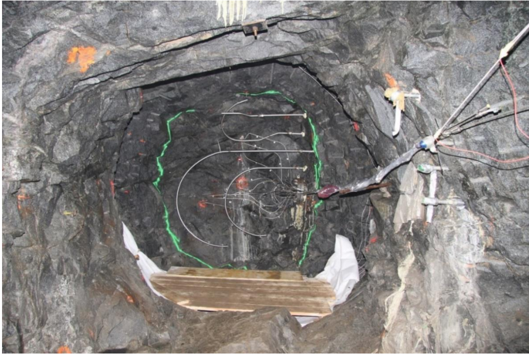
Figure 9 - Pressurisation chamber prepared for shotcreting (24 October 2014)
