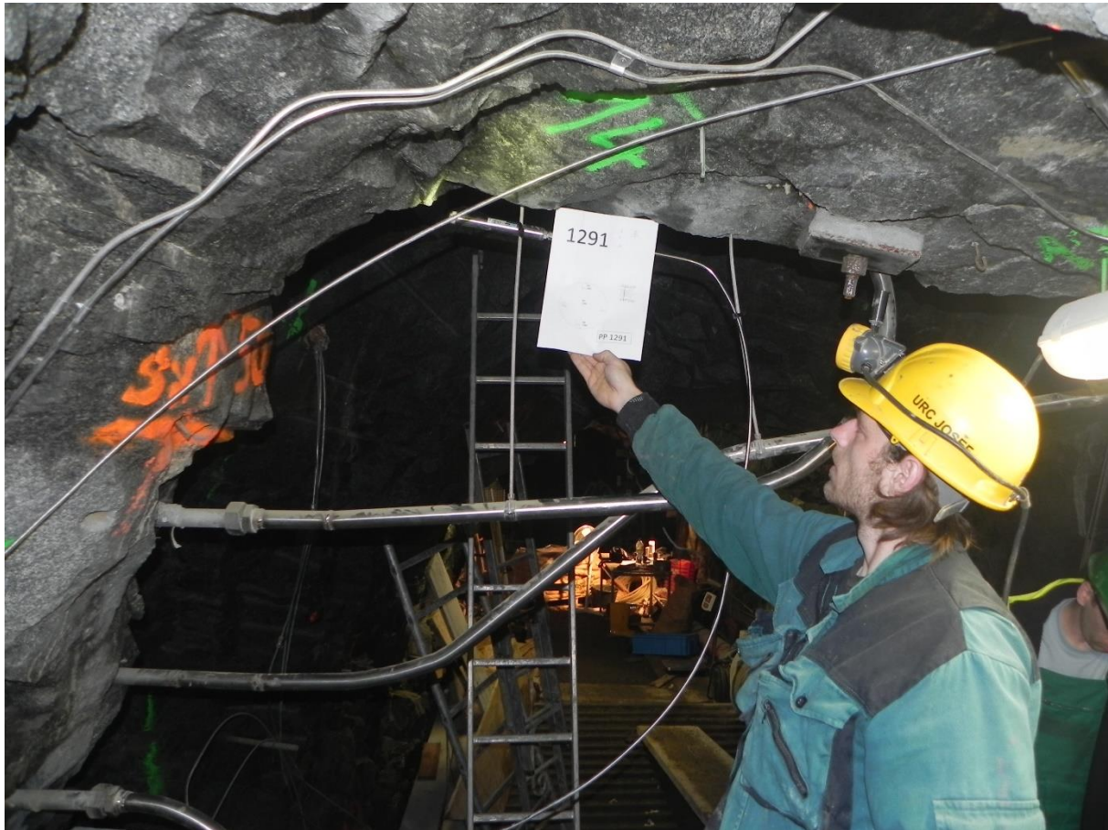
Figure 68 - Piezometer in the filter area
