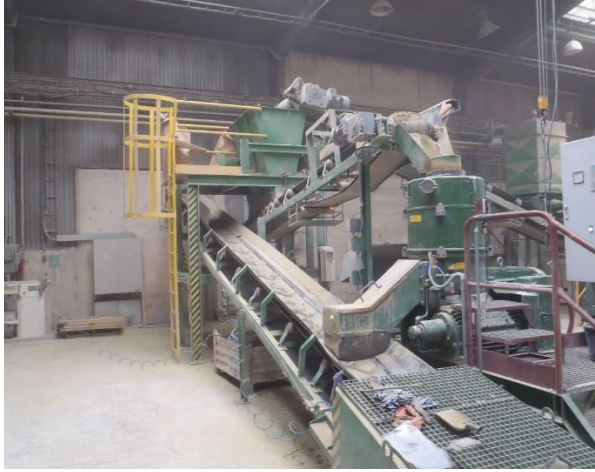
Figure 34 - Roller compaction machine
