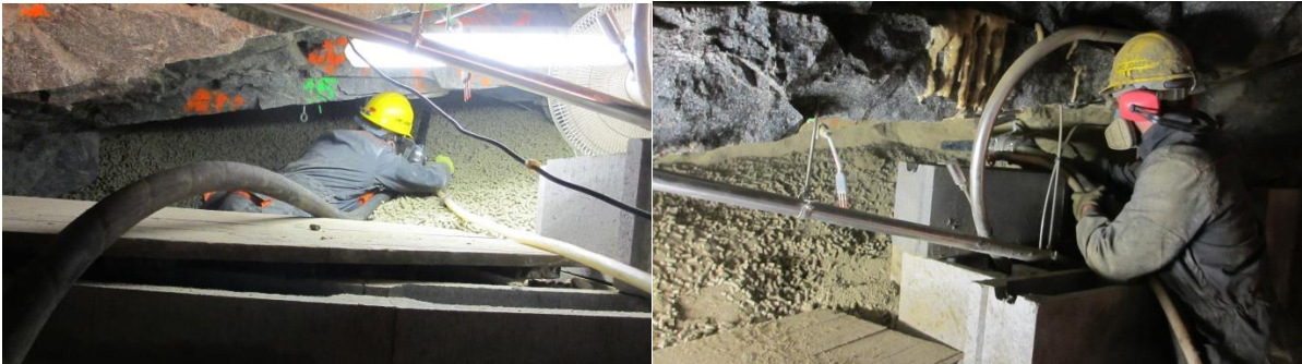
Figure 42 - Spraying of the bentonite
