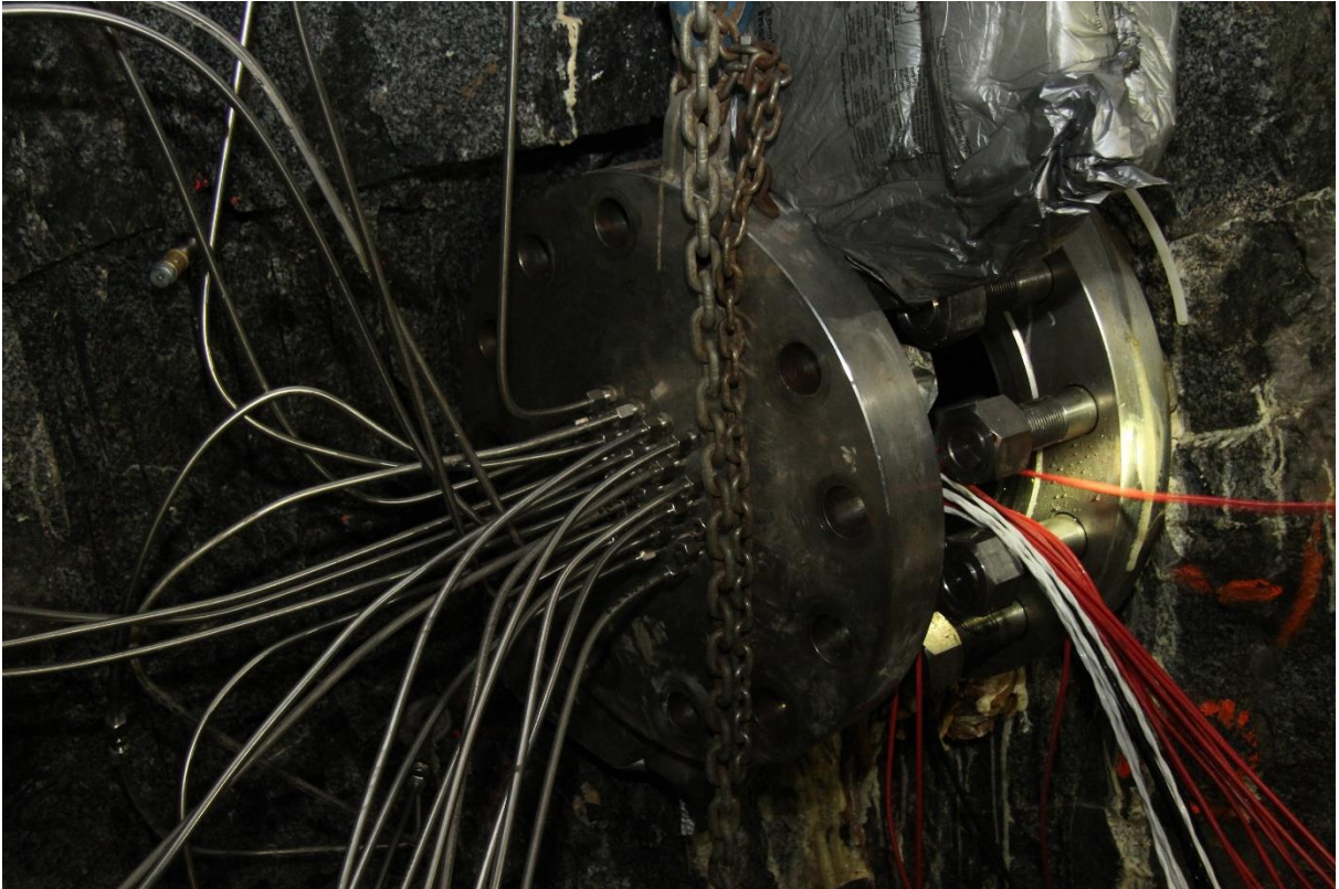
Figure 5 - Cable head before leading the cables through the borehole (29 August 2014)
