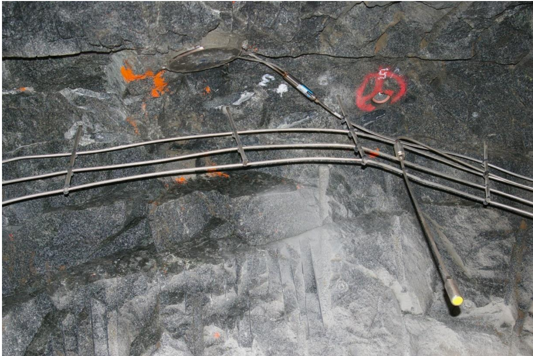
Figure 64 - Pressure cell on the rock face; cabling in protective tubing on “ladders”, thermometer
