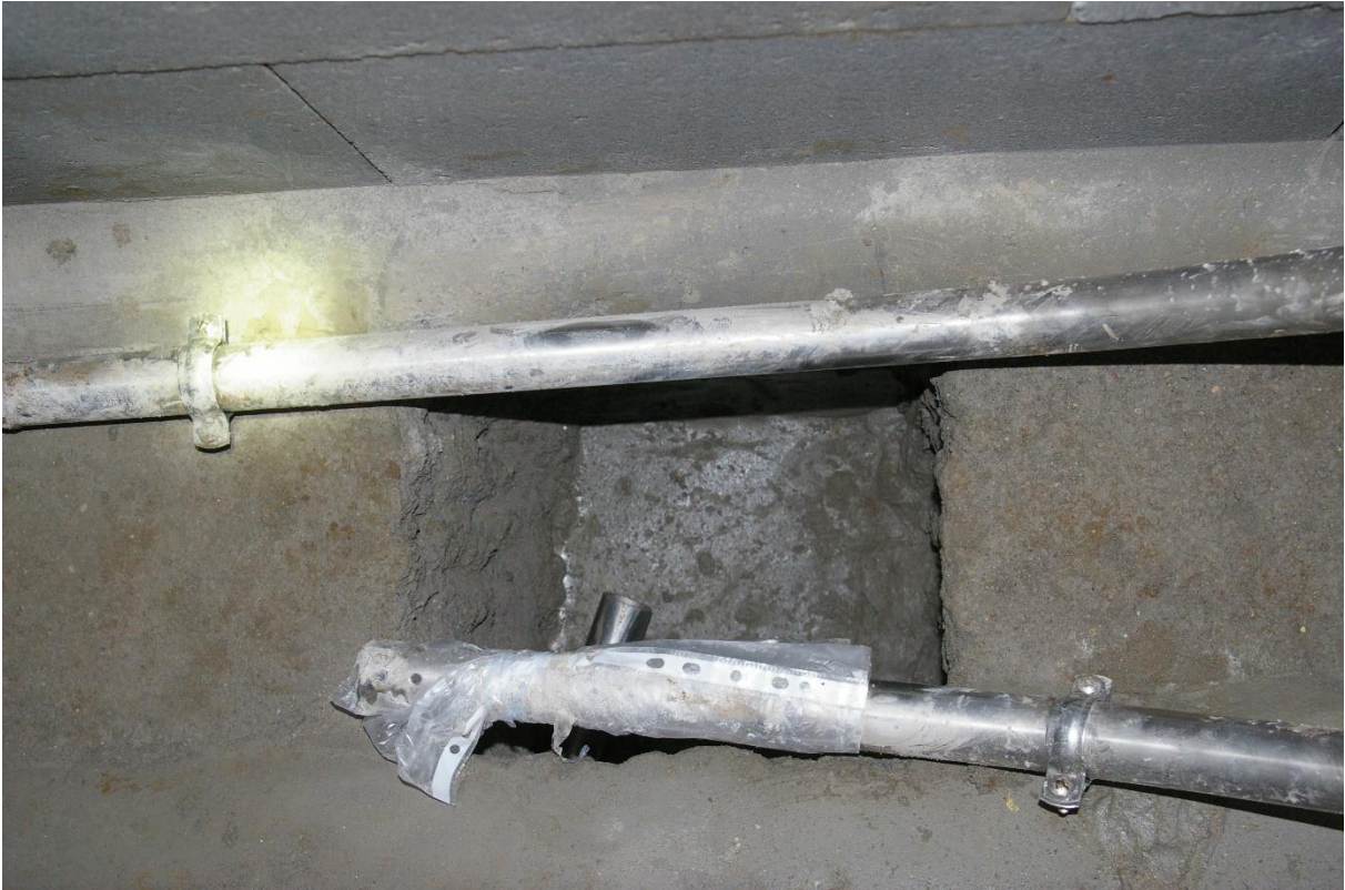
Figure 21 – Bottom drain of the filter (pressurisation tubes with temporary protection overlying the drain)
