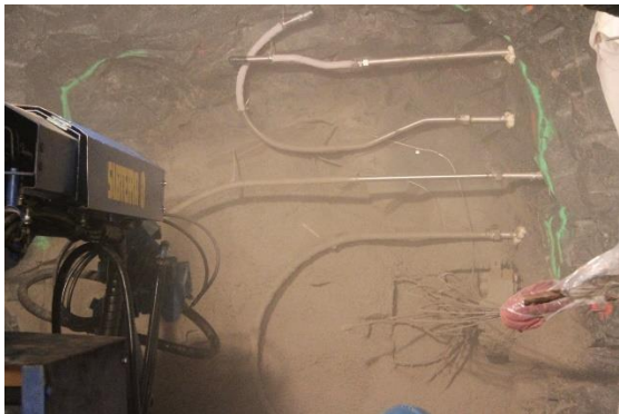
Figure 10 - Shotcreting of the chamber (27 October 2014)
