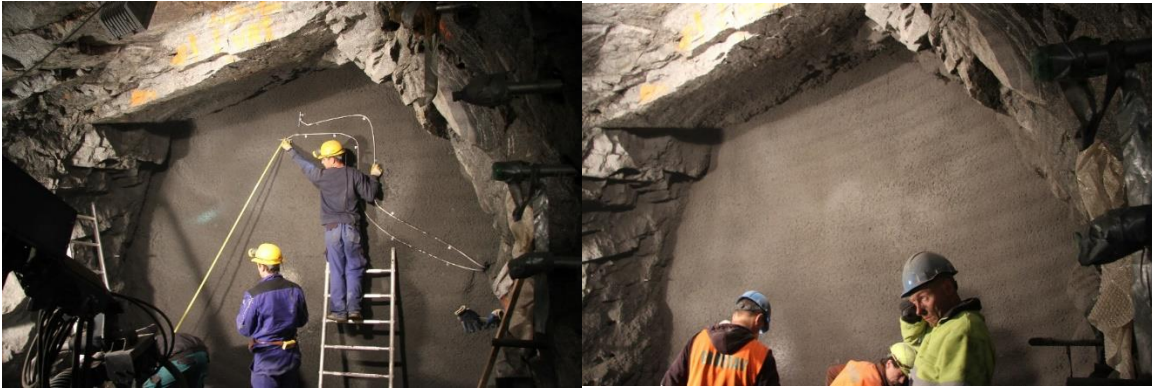
Figure 18 - Inner plug erection and sensor installation (12/13 December 2014) – reloading of the concrete mix, offloading the mix into the pump, shotcreting machine, first batches sprayed, instrumentation installation, finished plug
