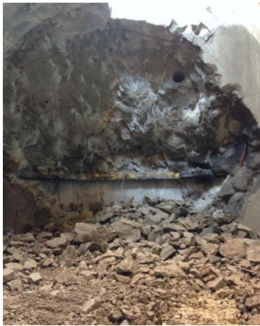
(c) Demolition of the low-pH shotcrete containment wall
