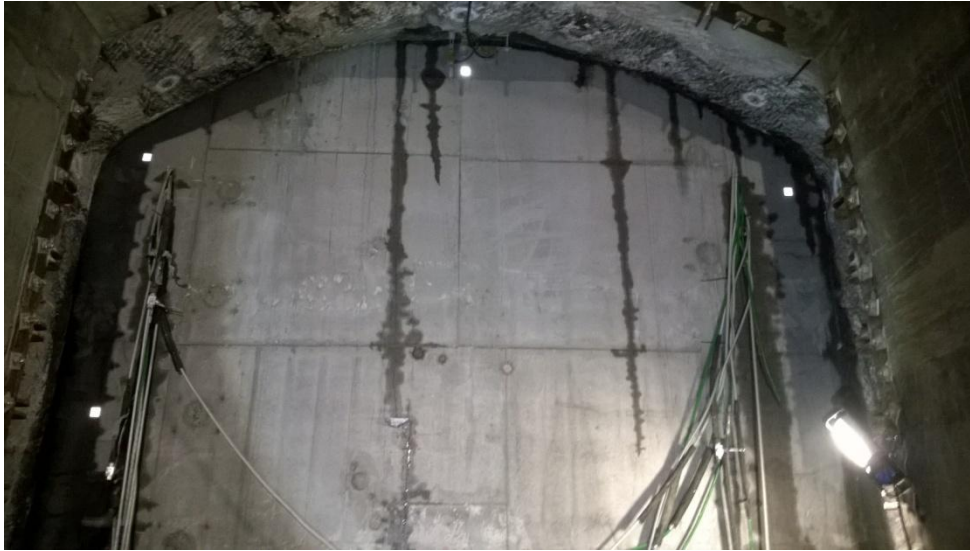
Figure 7.5: Visual appearance of minor plug leakage from the interface areas at top and sides of plug.
