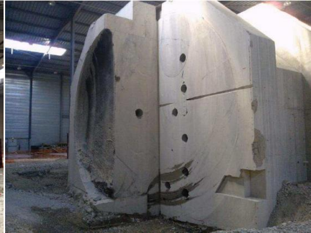
(b) Coring of the wire sawn low-pH shotcrete containment wall
