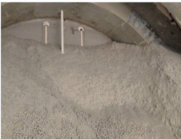
(e) Removal of the bentonite clay core
