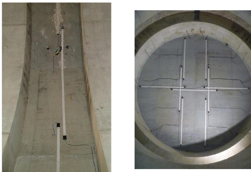
Figure 4.8: TDR sensors emplacement in a recess (left) and at front of SCC plug (right).
