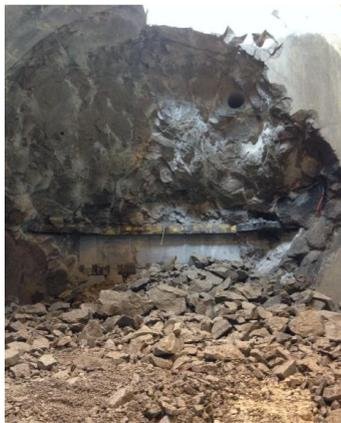
(c) Demolition of the low-pH shotcrete containment wall
