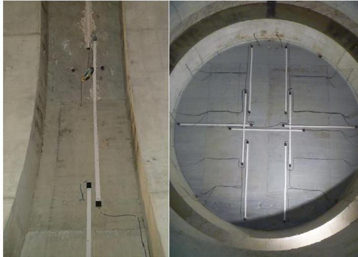
**Figure 2.8:** TDR sensors emplacement in a recess (left) and at front of SCC plug (right).
