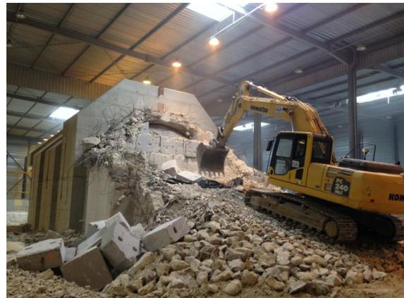
(d) Demolition of the low-pH SCC concrete containment wall
