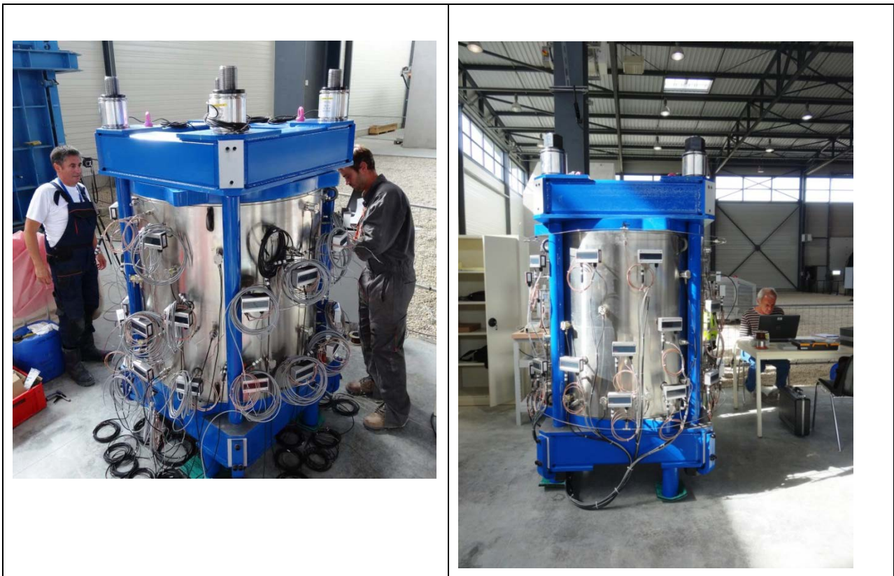
Figure 4-21 End of REM model installation with sensor cable connection and operational tests
