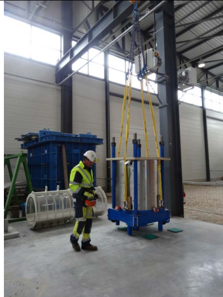
Installation of the vessel in its definitive location
