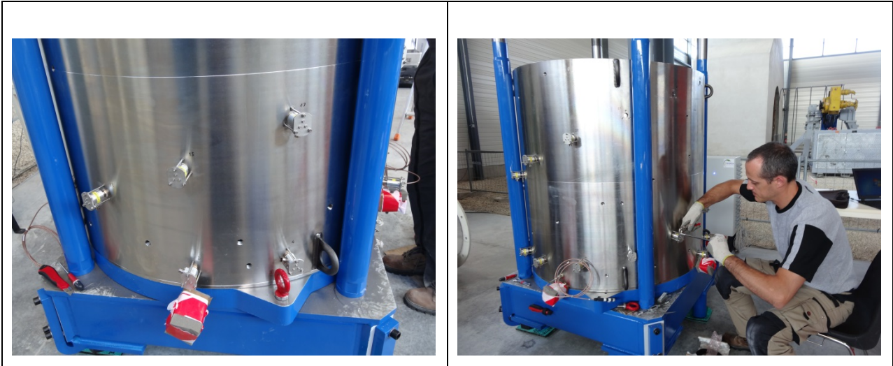
Figure 4-6 Installation of radial load cells
