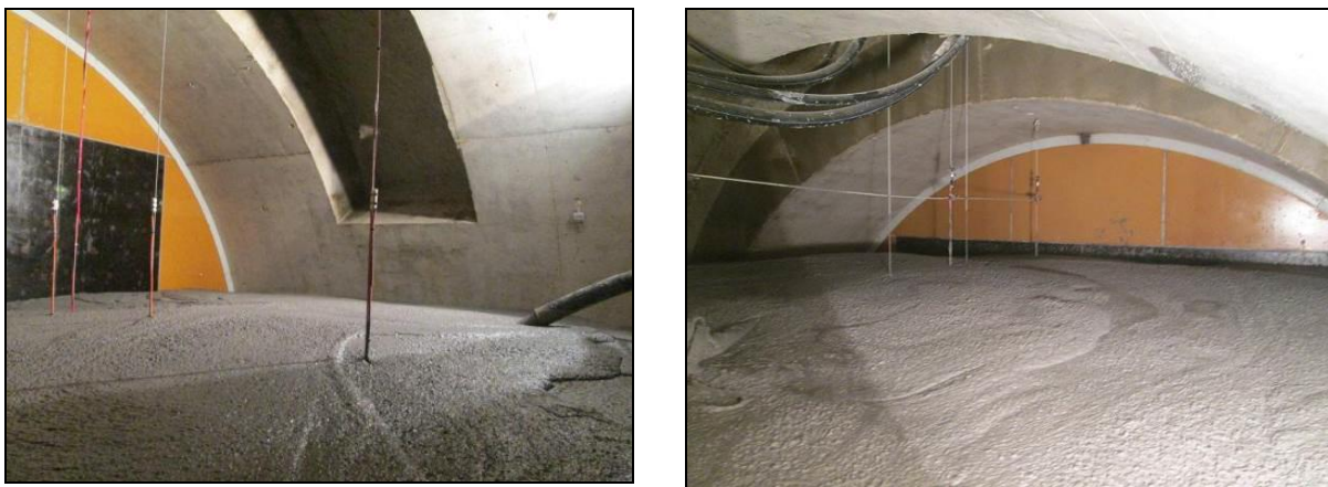
Figure 2.11: Pouring and even emplacement of SCC inside the test box (left) and emplacement of SCC close to the recess (right) (D3.8, Bosgiraud et al. , 2014).
