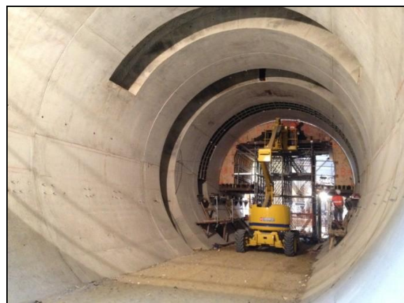
f) The completed test box
