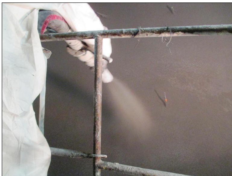
Figure 2.17: Installing the second containment wall made of low pH shotcrete in FSS.
