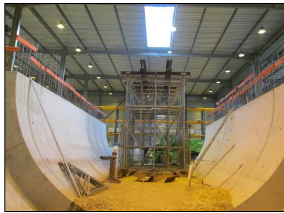
d) The completed lower part of the test box with a sand layer at the bottom and scaffolding also shown
