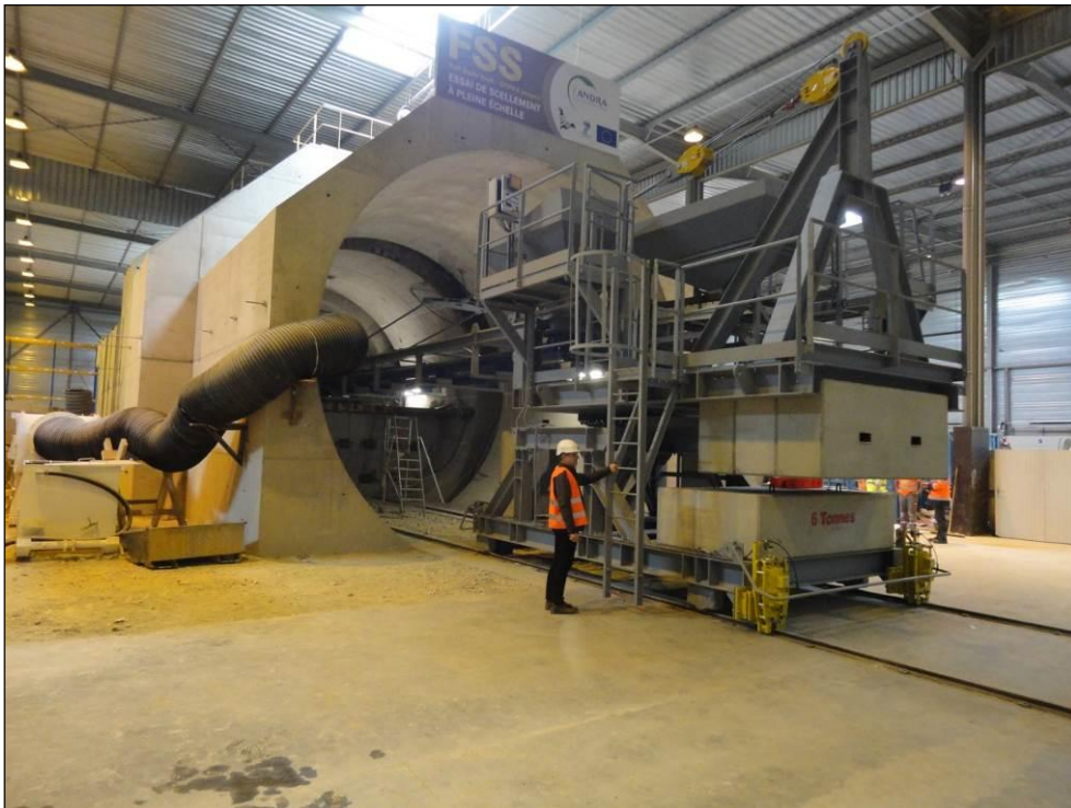
Figure 2.13: The bentonite mix emplacement machine.
