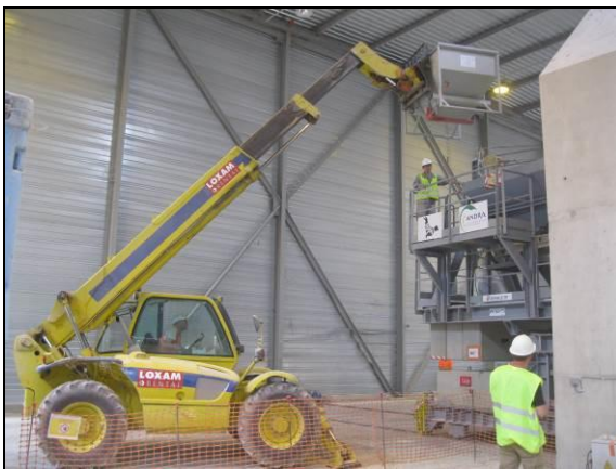
Figure 2.14: Emptying of an octabin containing bentonite pellets (left) and a big bag with bentonite powder (right) into hoppers.
