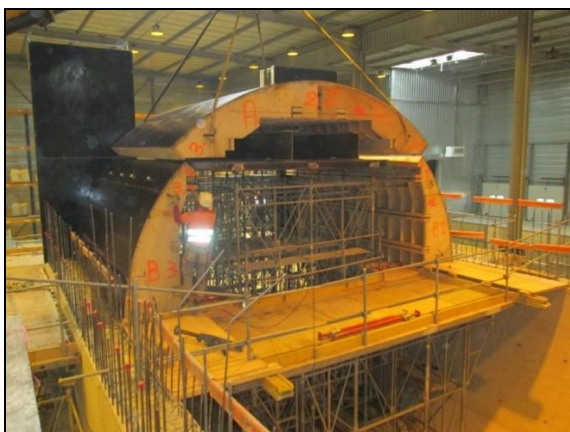
e) Removal and translation of the wooden formwork between the two phases of the upper block casting
