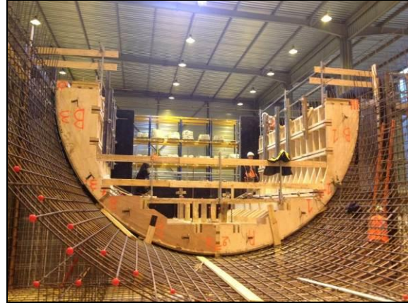
b) The inner wooden form and steel form
