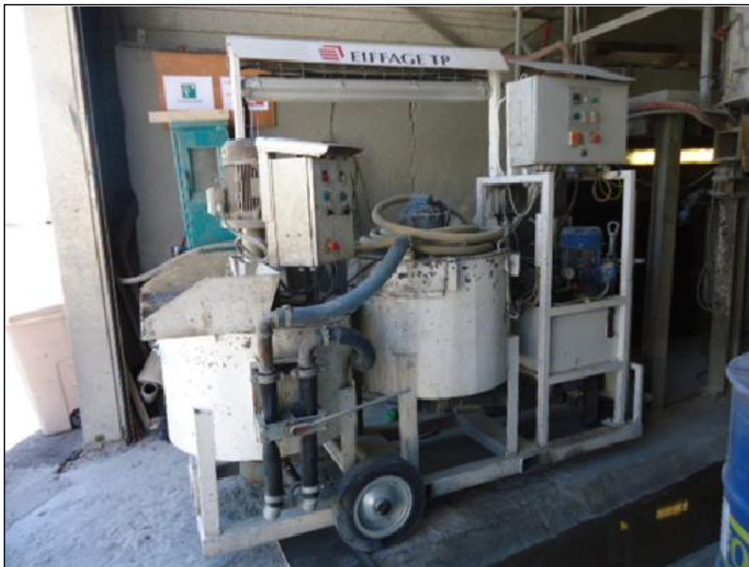
Figure 2.12: Grouting machine used for bonding in the FSS experiment.
