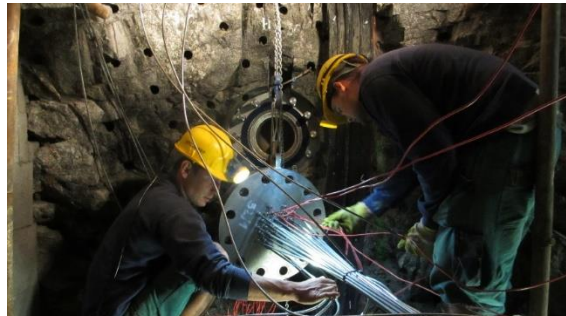
Figure 7 - Cable head preparation
