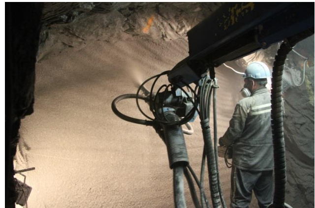
Figure 4. Shotcrete of EPSP plug.
