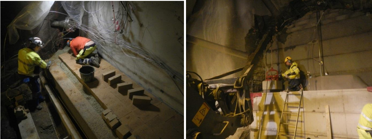
Figure 2. Installation of backfill blocks behind Leca beams (left) and seal blocks behind concrete beams (right).
