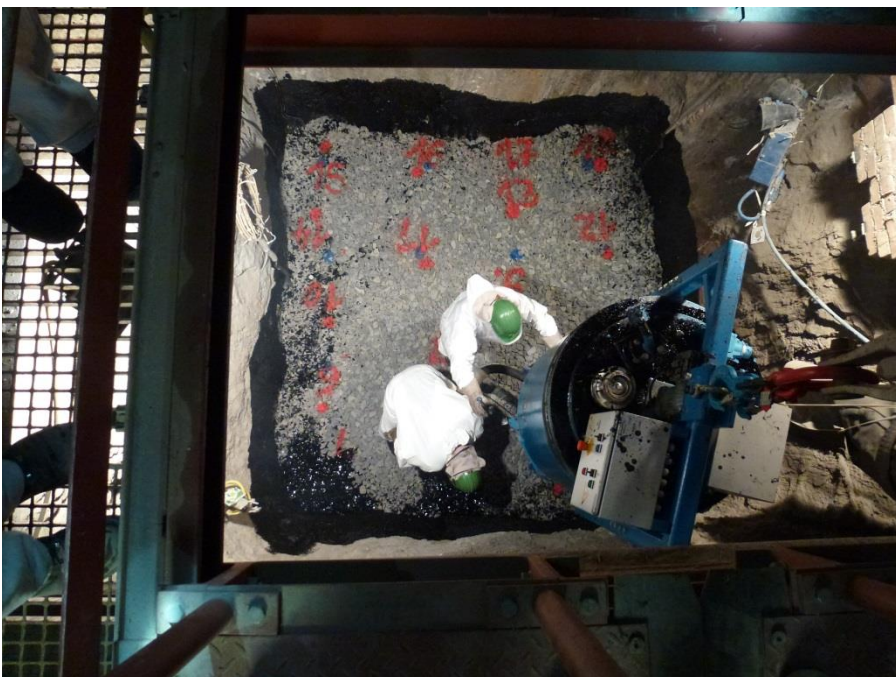
Fig. 4: Filling in the hot asphalt
