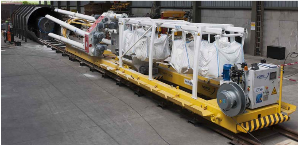
Figure 3: Photo of the rear end of the backfilling machine ready to start backfilling the steel tunnel tube
