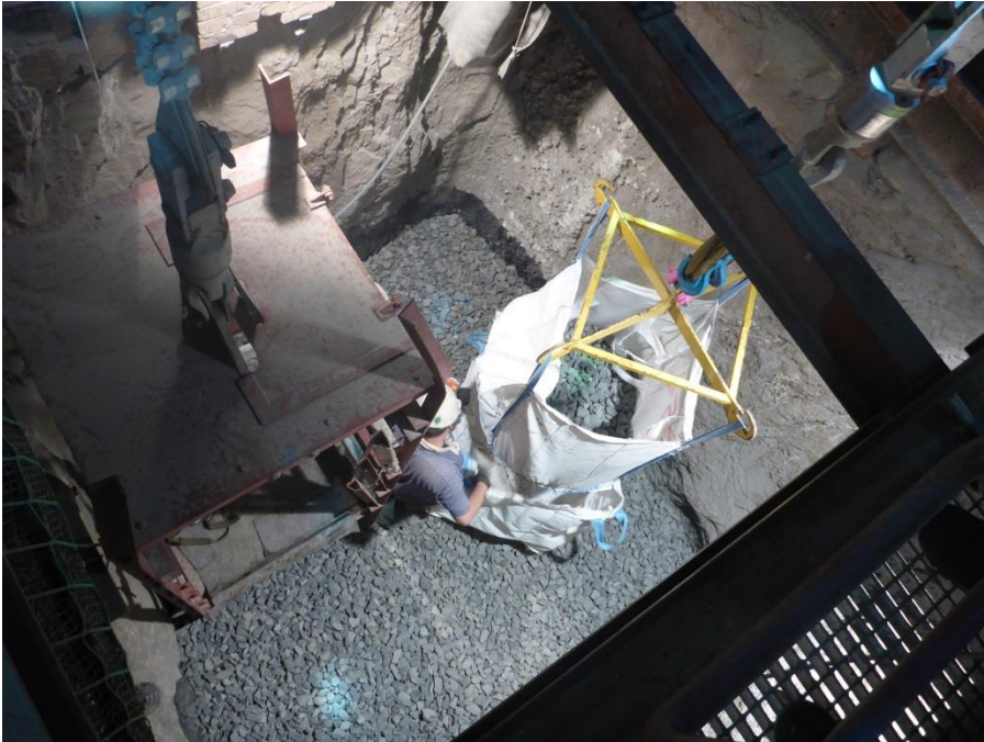
Fig. 3: Transportation of the gravel in the blind shaft
