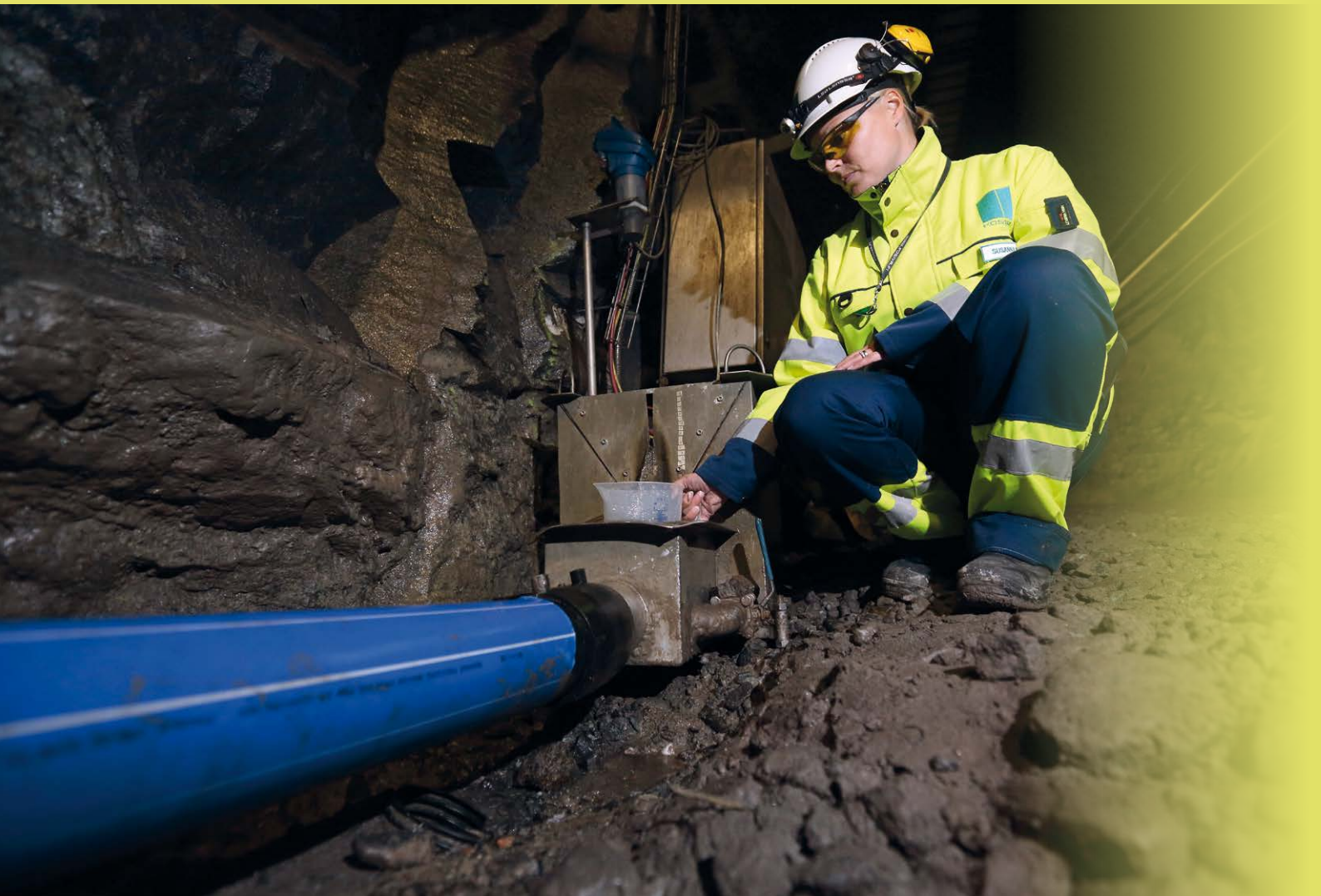
The quantity and quality of leakage from the bedrock to ONKALO is monitored on a regular basis.
