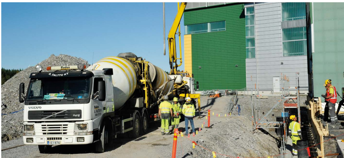
A view of the construction site of the second phase of the lifting equipment building in September.
