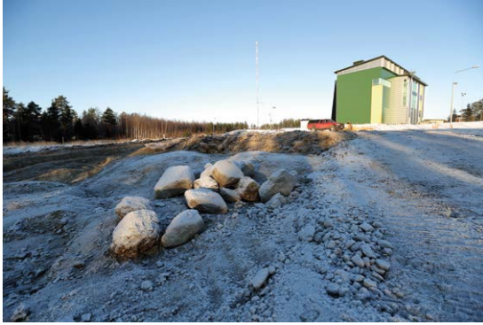
Area works proceed on the future plant site of the final disposal repository.
