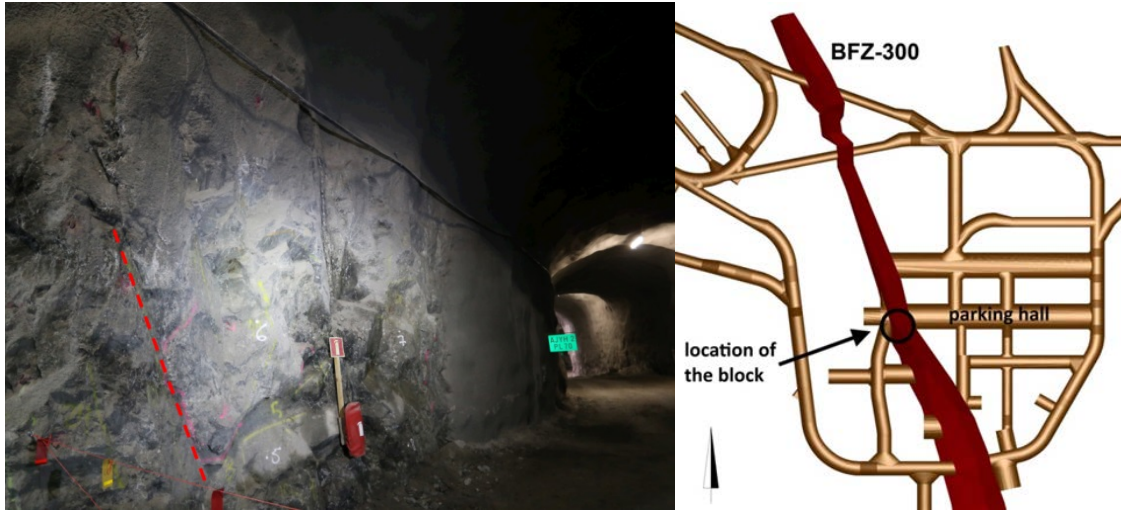
Figure 2-2. Test area before the experiment (right) and the location of the test block (left). The loose block is delimited by a fracture on its left side (red dashed line).
