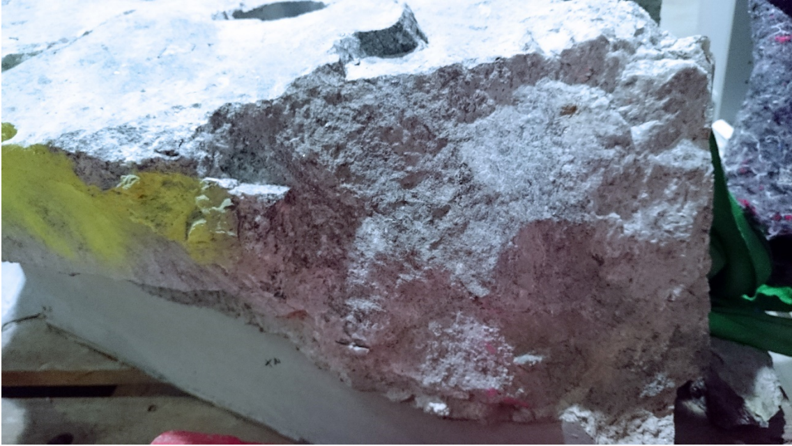
Figure 4-5. The upper left corner of the block.
