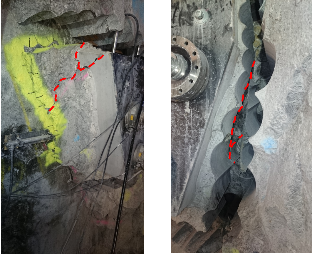
Figure 4-3. Observed breakages after test execution. The upper left corner broke (left) and part of the right edge broke (right). See also Figure 4-3.
